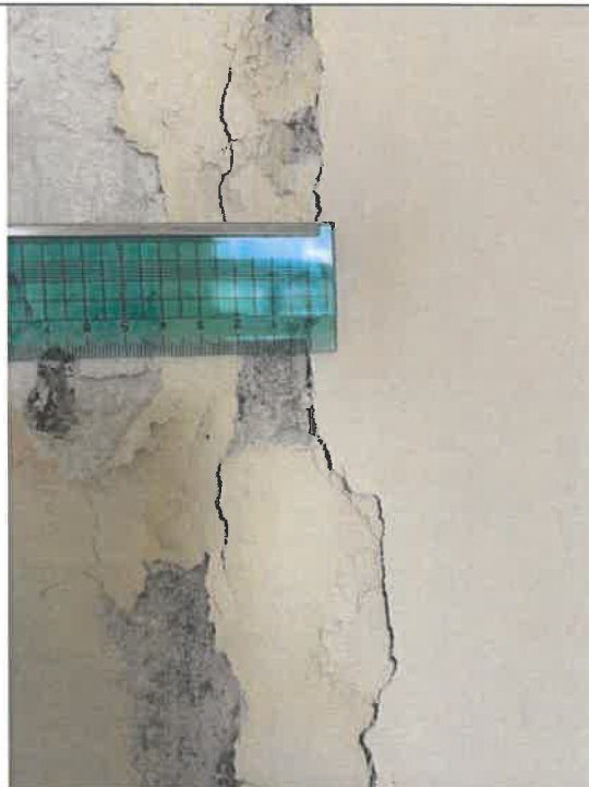
Photo: G303-38: Fine Crack on Surface
