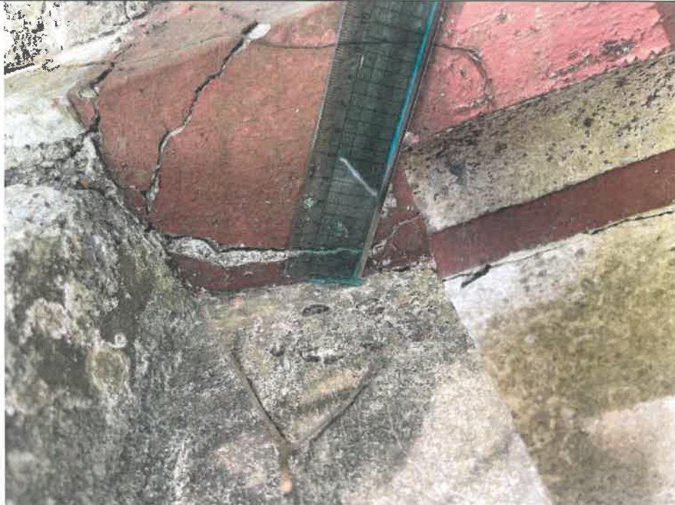
Photo : G202-13 Wide Crack on Surface
