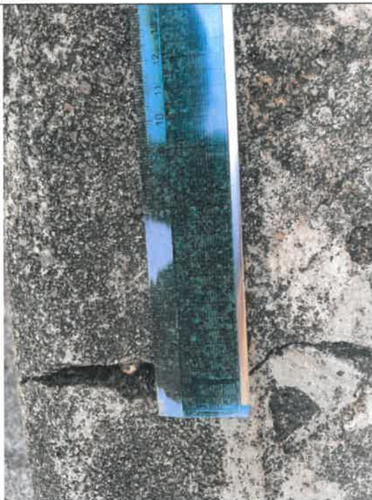
Photo G308-33: Wide Crack
