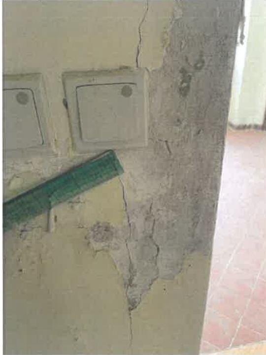
Photo: G303-37: Fine Crack on Surface
