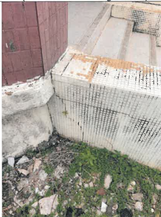
Photo: G303-39: Moderate Crack on Surface
