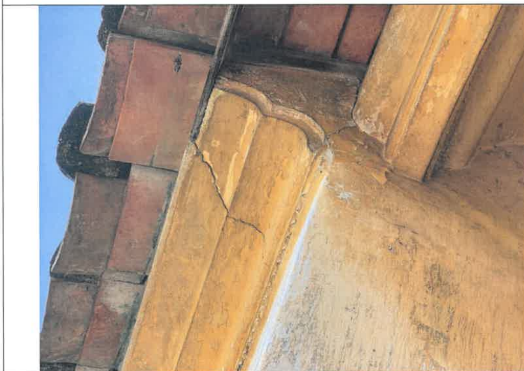
Photo G308-38: Wide Crack
