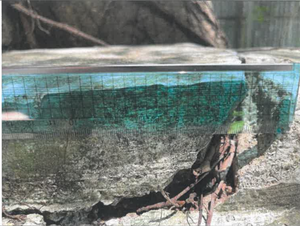
Photo : G202-17 Wide Crack on Surface
