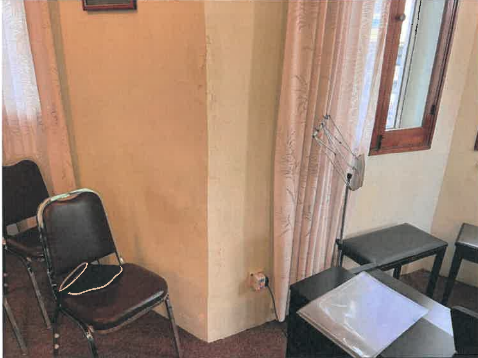
Photo: HKT03-23 Peel off paint with moisture
