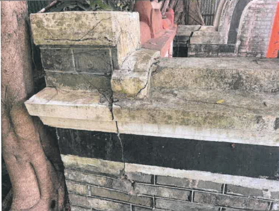
Photo : G202-19 Moderate Crack on Surface
