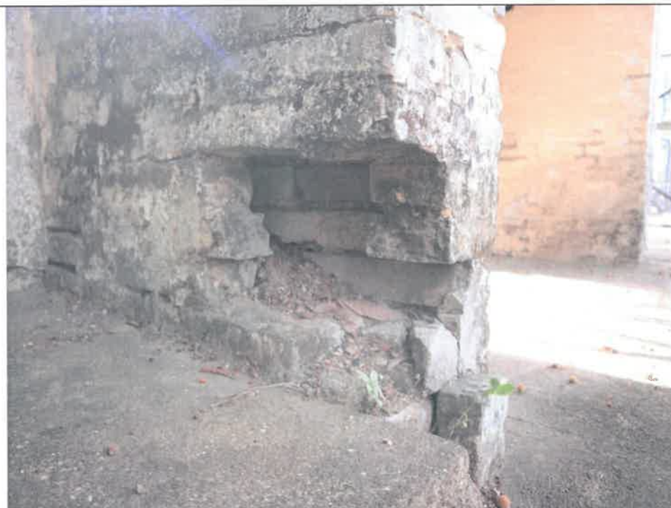
Photo 1-EG-10 Missing bricks on the structure
