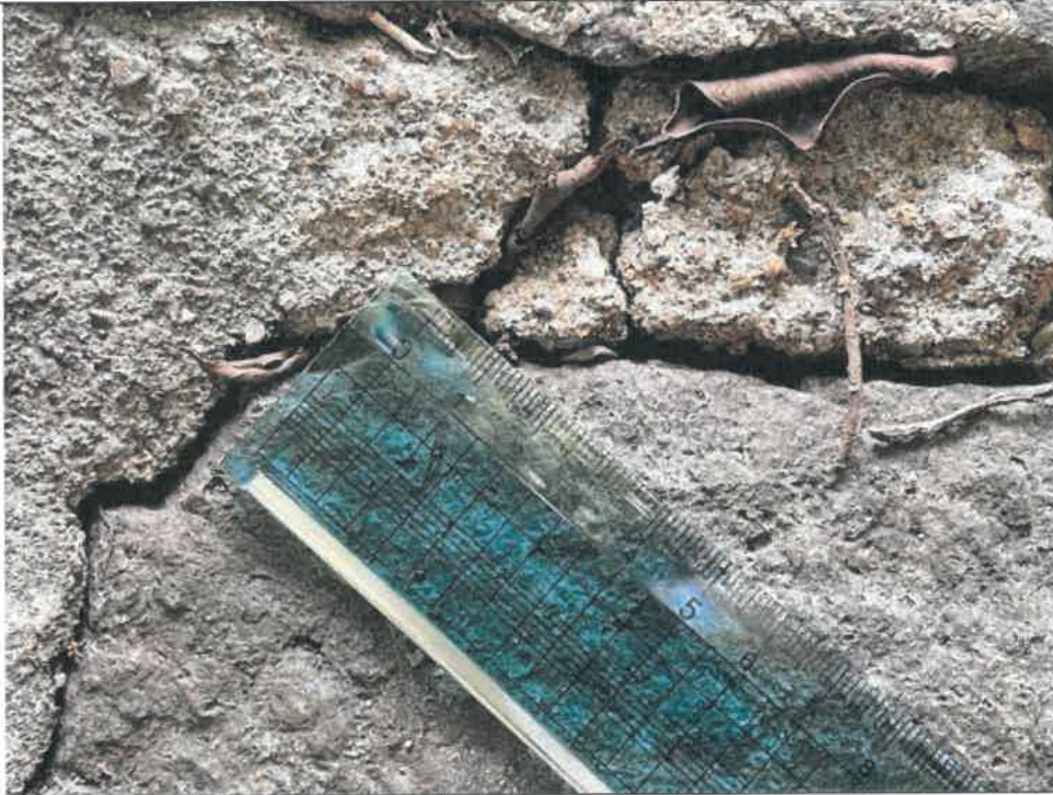
Photo : G202-11 Wide Crack on Surface
