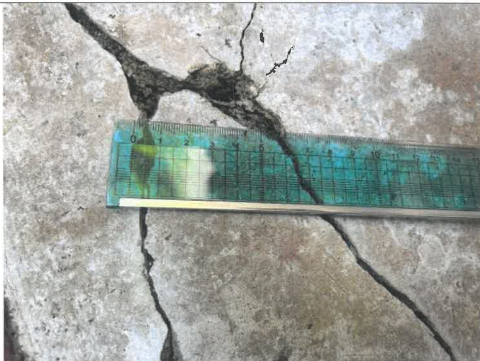
Photo : G202-14 Wide Crack on Surface
