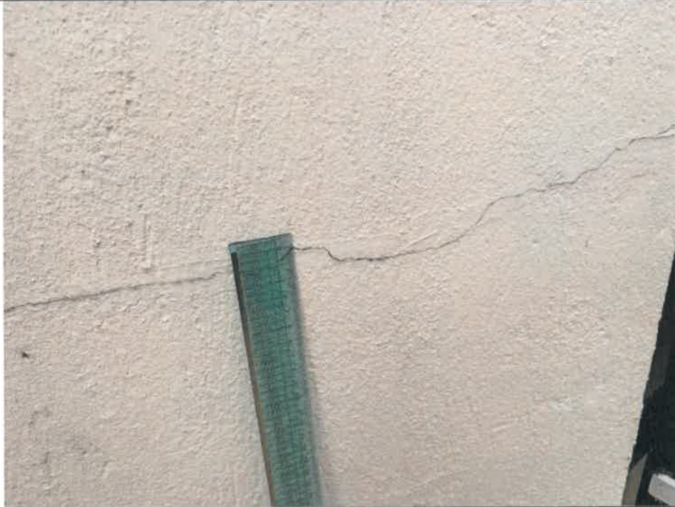
Photo: G303-35: Fine Crack on Surface
