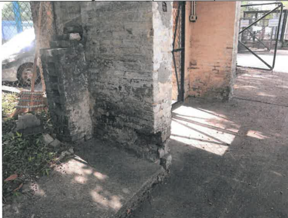
Photo 1- EG-9: Missing bricks on the structure
