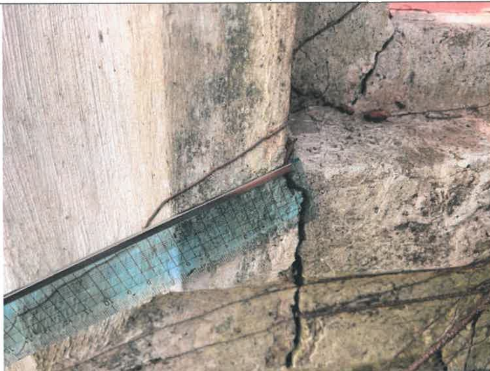
Photo : G202-15 Wide Crack on Surface
