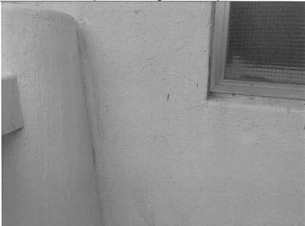
Photo: HKT03-53 Fine cracks on surface
