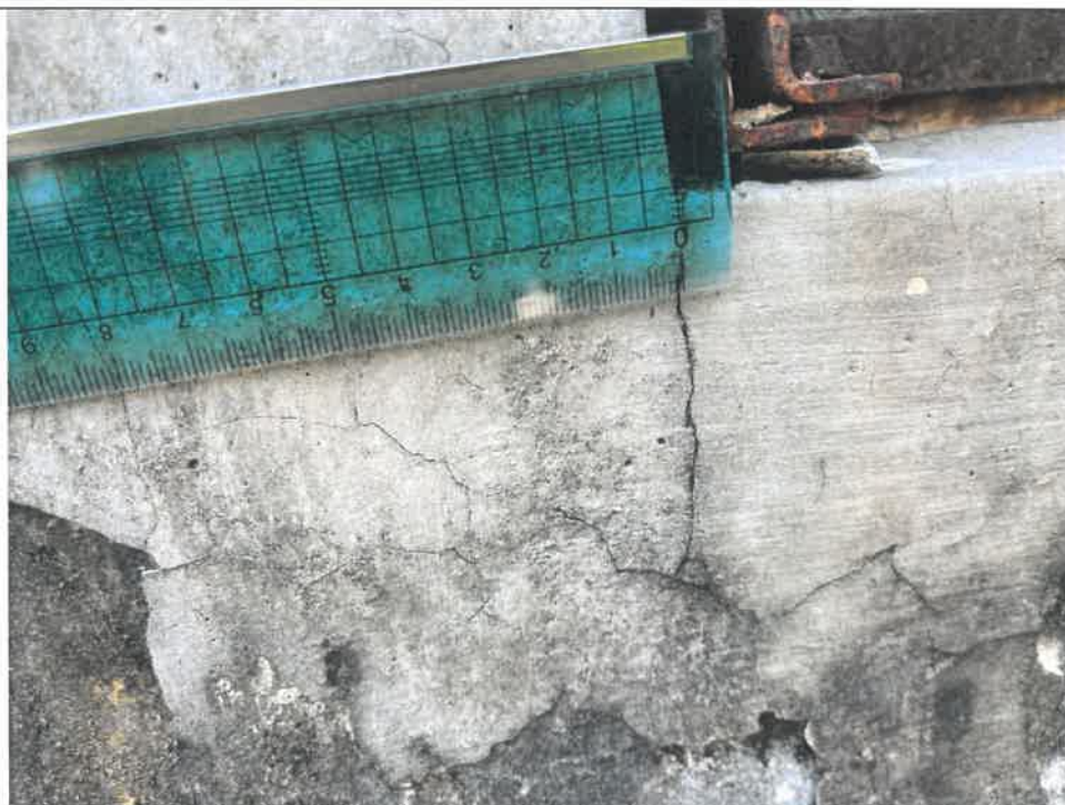
Photo G308-28: Moderate Crack
