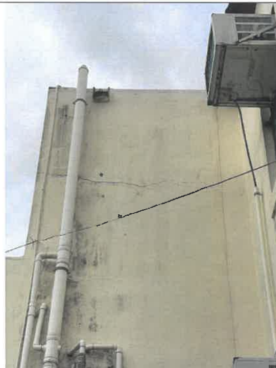
Photo: G303-42: Moderate Crack on Surface
