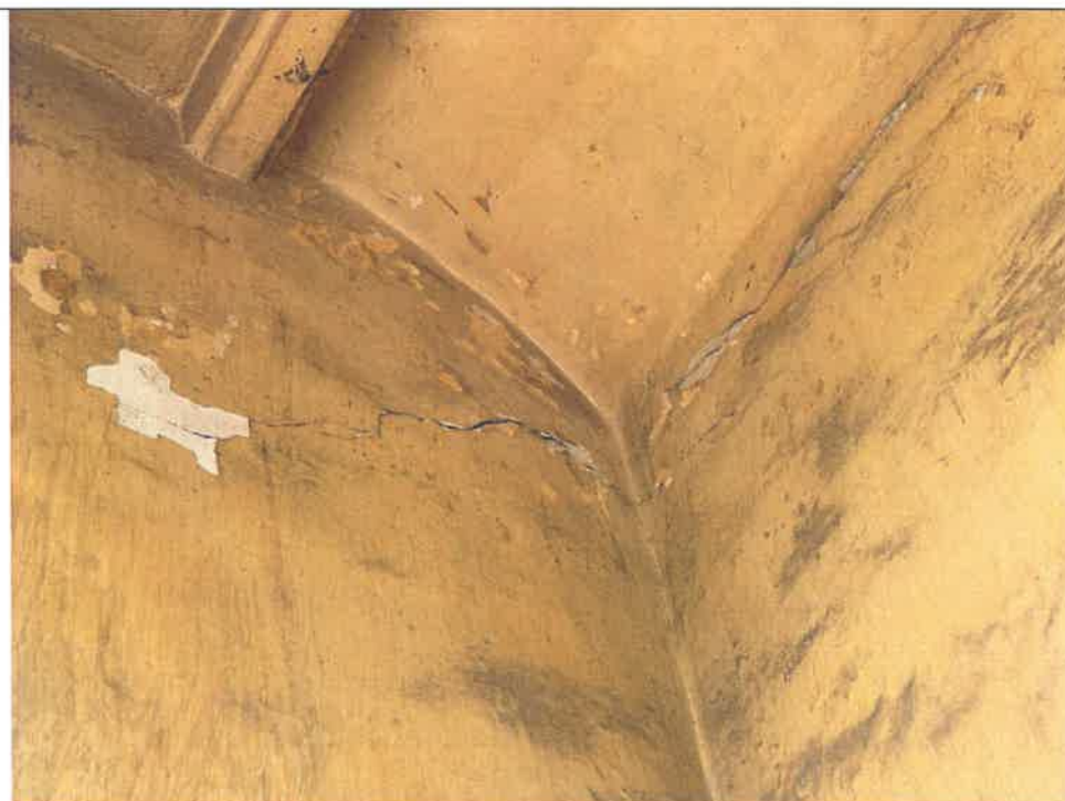
Photo G308-36: Moderate Crack on Surface
