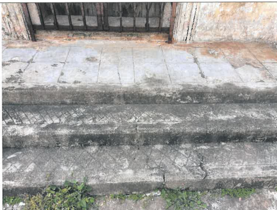
Photo G308-34: Wide Crack
