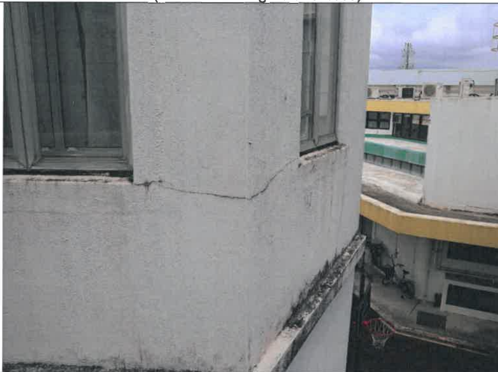
Photo: HKT03-51 Moderate cracks on surface
