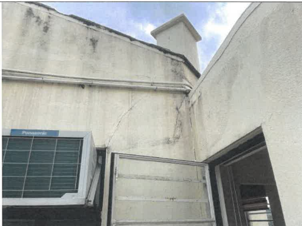
Photo: G303-34: Fine Crack on Surface
