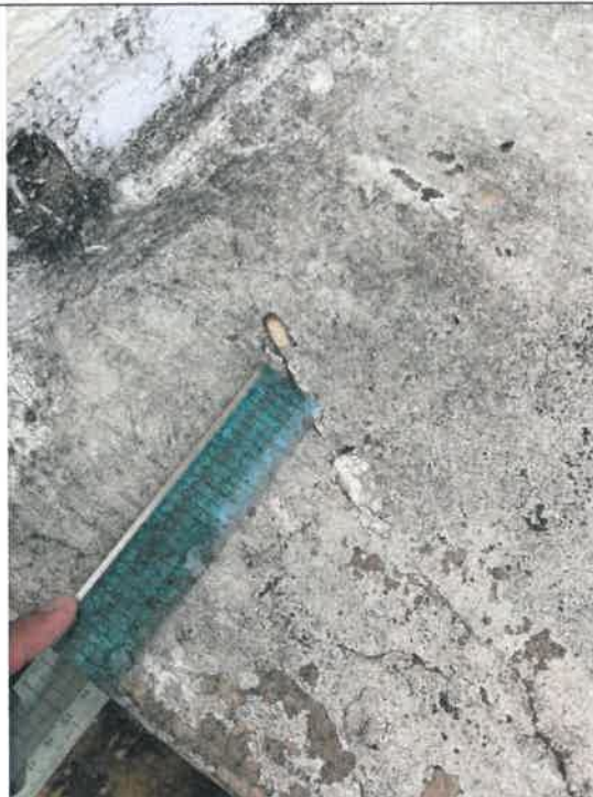
Photo: G303-36: Fine Crack on Surface
