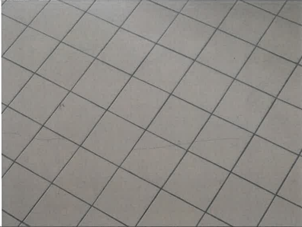
Photo: HKT03-33 Crack on floor tiles
