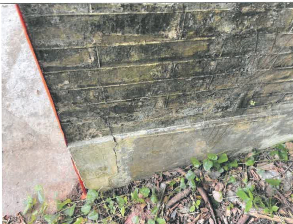
Photo : G202-16 Fine Crack on Surface
