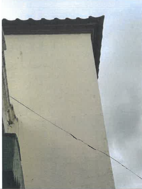
Photo: G303-41: Fine Crack on Surface
