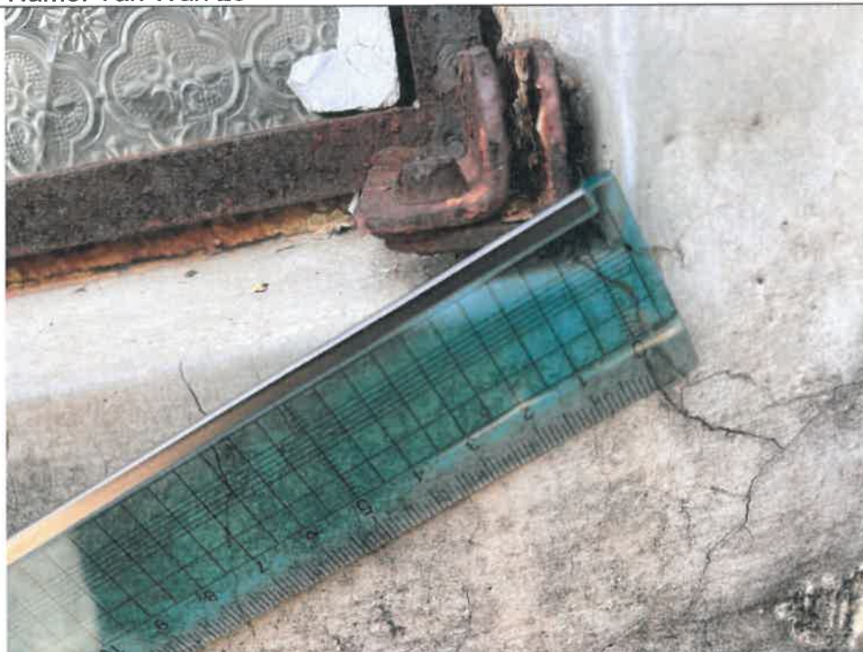
Photo G308-29: Moderate Crack
