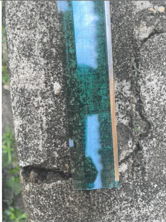
Photo G308-31: Wide Crack
