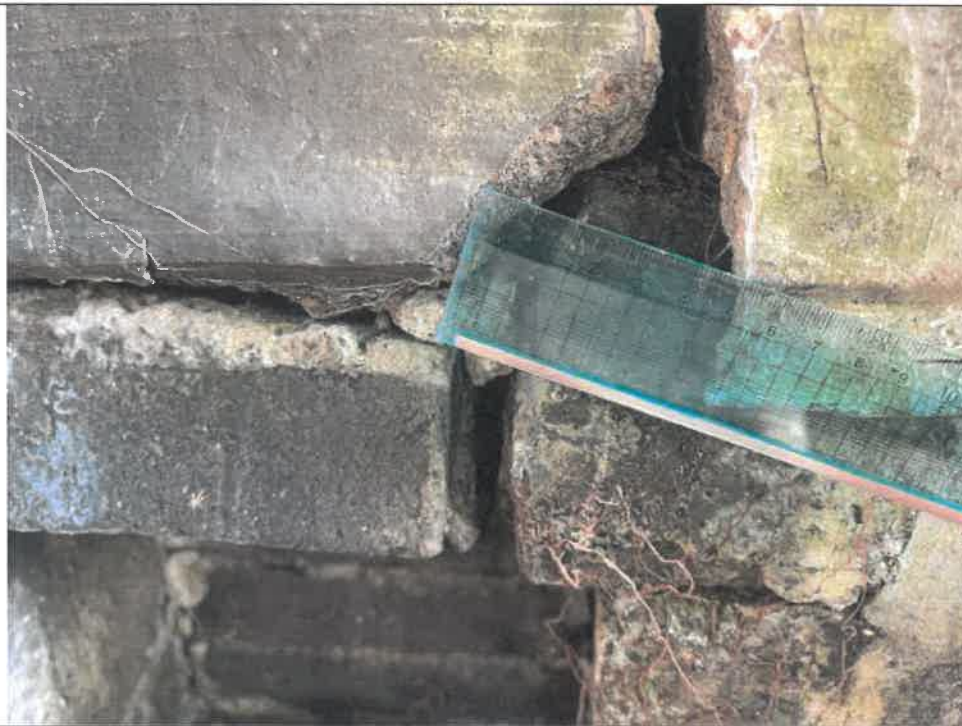
Photo : G202-18 Wide Crack on Surface
