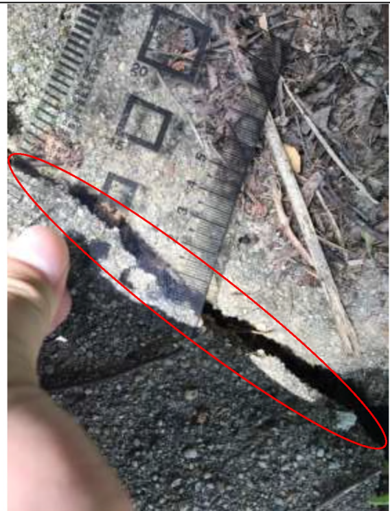
3A-D15(1) – Wide Crack on Slope (Length:600mm/Width:5.00mm)
