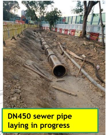
**DN450 sewer pipe laying in progress**
