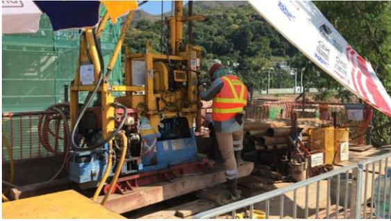
Predrilling for tower crane foundation next to E2-02
