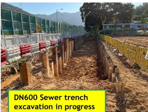
**DN600 Sewer trench excavation in progress**
