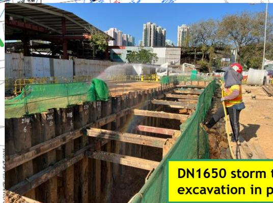
**DN1650 storm trench excavation in progress**
