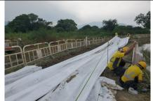
Laying geotextile under rock layer to allow effective reinstatement of temporary access road
