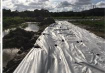
Laying geotextile under rock layer to allow effective reinstatement of temporary access road
