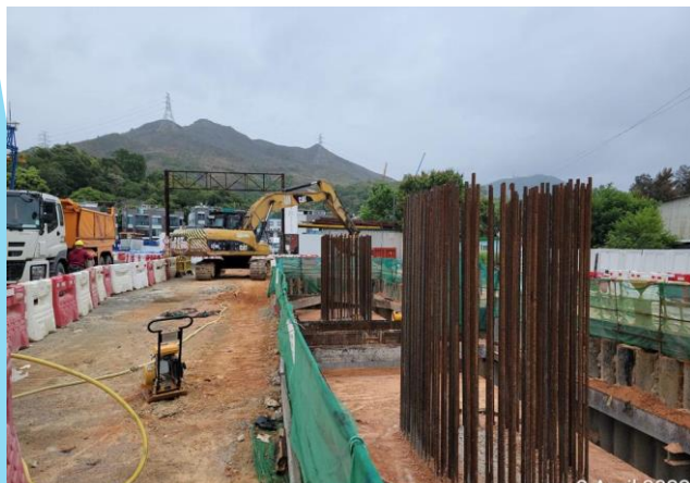
D1-01/ E1-01 Pile Cap cast on 15/3/22. Backfilling in Progress.
