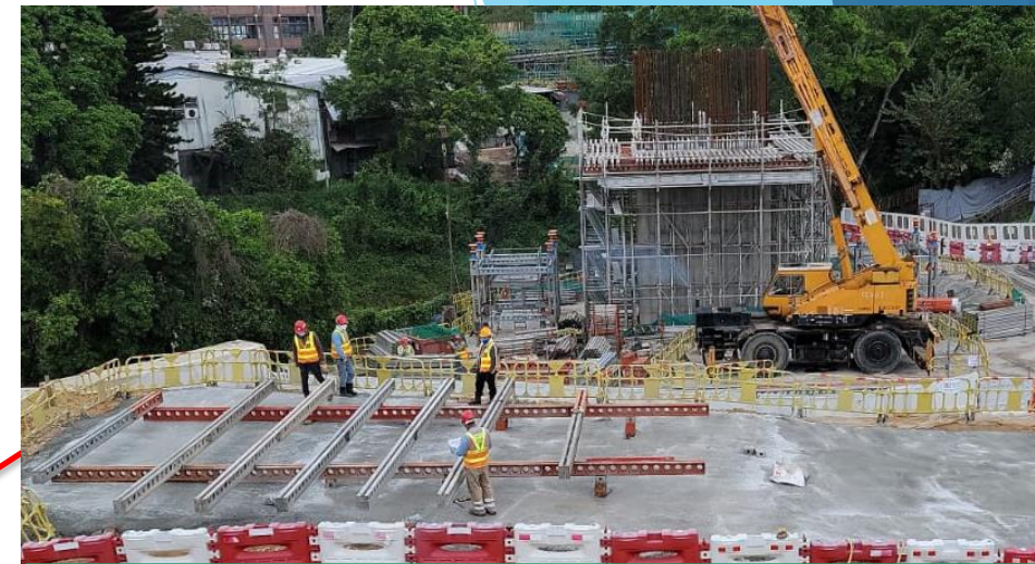
Falsework erection in progress for C4-03 Cross Head Construction.
