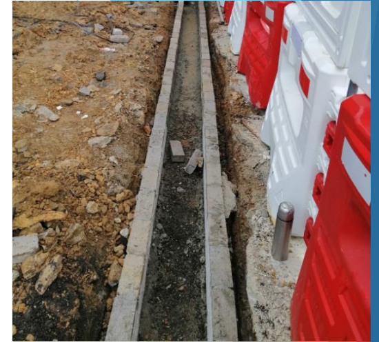
Temporary drainage in progress
