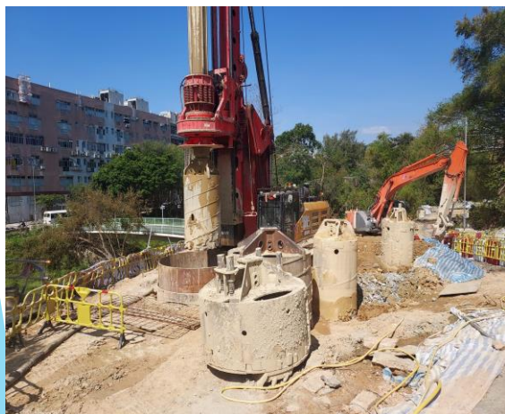
C3-02-P1 Bored Pile completed C3-02-P2 in progress
