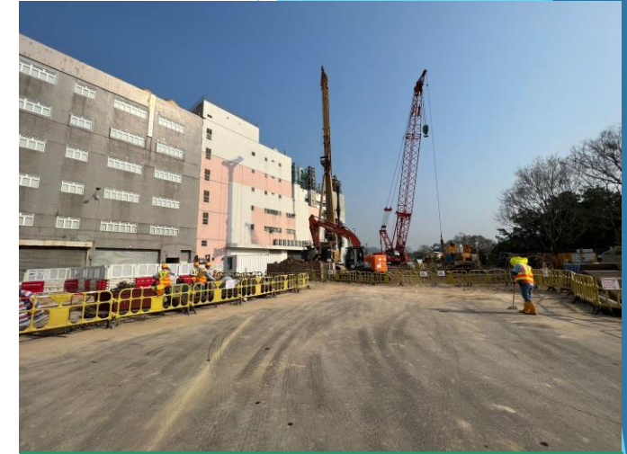
Bored pile works in C1-03
