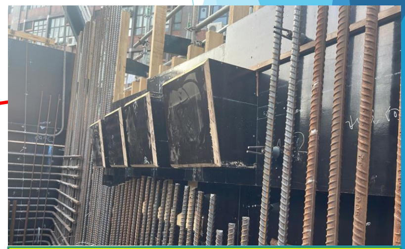
Formwork erection and rebar fixing at C4-01 Portal Beam Construction in progress
