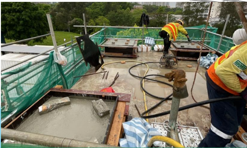
C4-04bM bearing plinths completed
