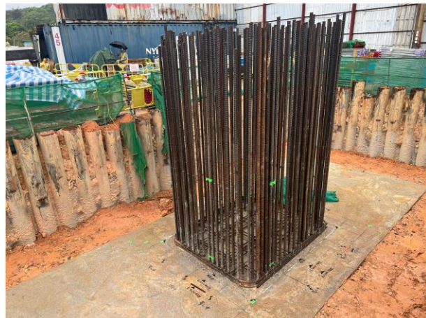
E1-02 Pier kicker construction in progress
