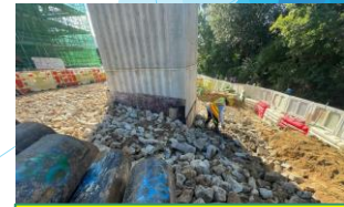
D1-04 backfilling and pipe pile extraction. Handover to Viaduct Team on 09/12/22
