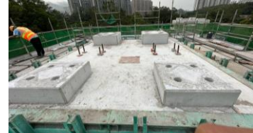
E1-04 bearing plinth completed on 20/11/22
