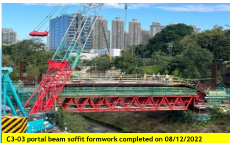
C3-03 portal beam soffit formwork completed on 08/12/22
