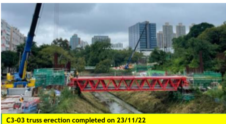
C3-03 truss erection completed on 23/11/22
