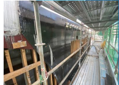
C4-02 Dismantling of formwork & falsework in progress
