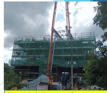
Concreting for C4-02 cross head (1 st pour) completed on 11/11/2022
