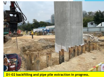
D1-02 backfilling and pipe pile extraction in progress.
