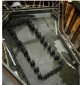
B1-02b Pile Cap Concreted
