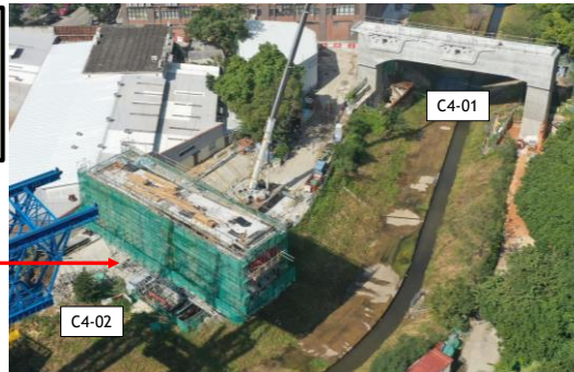
C4-02 Dismantling of formwork & falsework in progress
