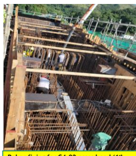
Rebar fixing for C4-02 cross head (1 st pour) completed on 10/11/2022
