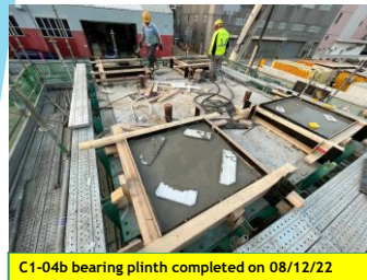
C1-04b bearing plinth completed on 08/12/22
