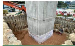
E1-04 backfilling and pipe pile extraction in progress.
