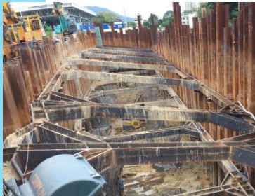
B1-01M 3 rd layer excavation in progress
