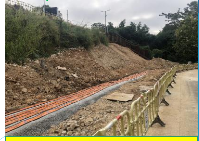
CLP installation of spare duct at Ch. 0 - 50 commenced on 23/11/2022
