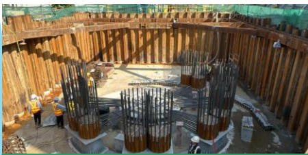
E2-01 reaction blocks complete concreting on 03/12/22. Installation of stanchion and sand box completed on 10/12/22.
