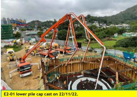
E2-01 lower pile cap cast on 22/11/22.
