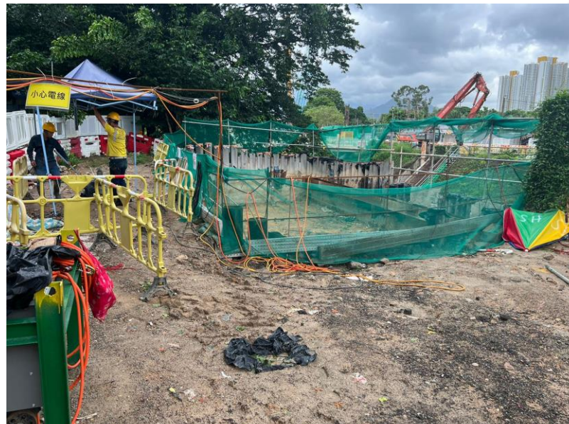
C1-01b 1 st layer of waling and struts
