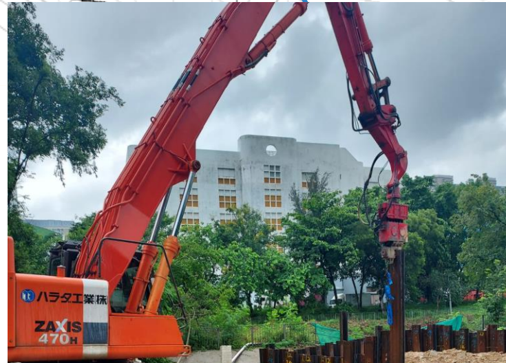
C2-02 sheet piling in progress
