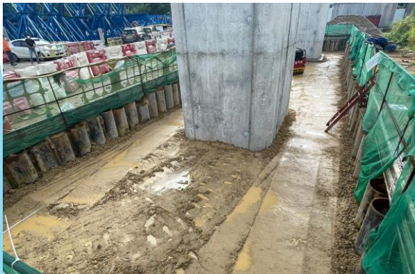
D1-01/ E1-01 Column completed Backfilling in Progress.
