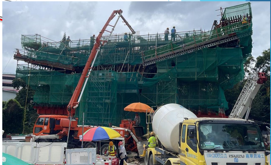
Concreting of C4-03 Cross Head (1st pour) on 20/06/22
