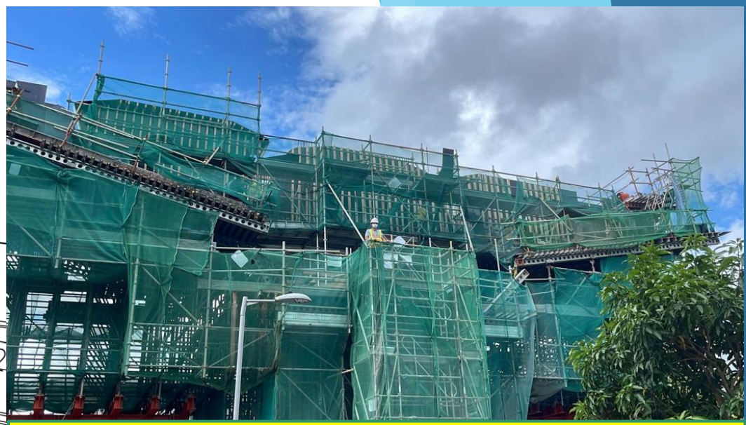
Timber formwork erection for C4-03 Cross Head (2nd Pour) completed
