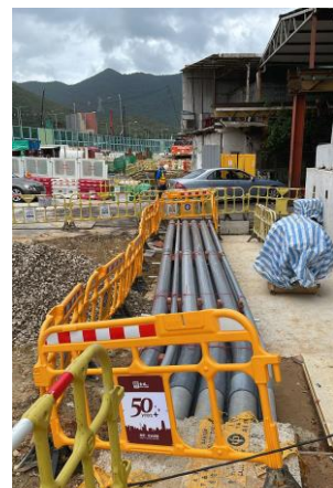
CLP 132 & 11kv ducting
