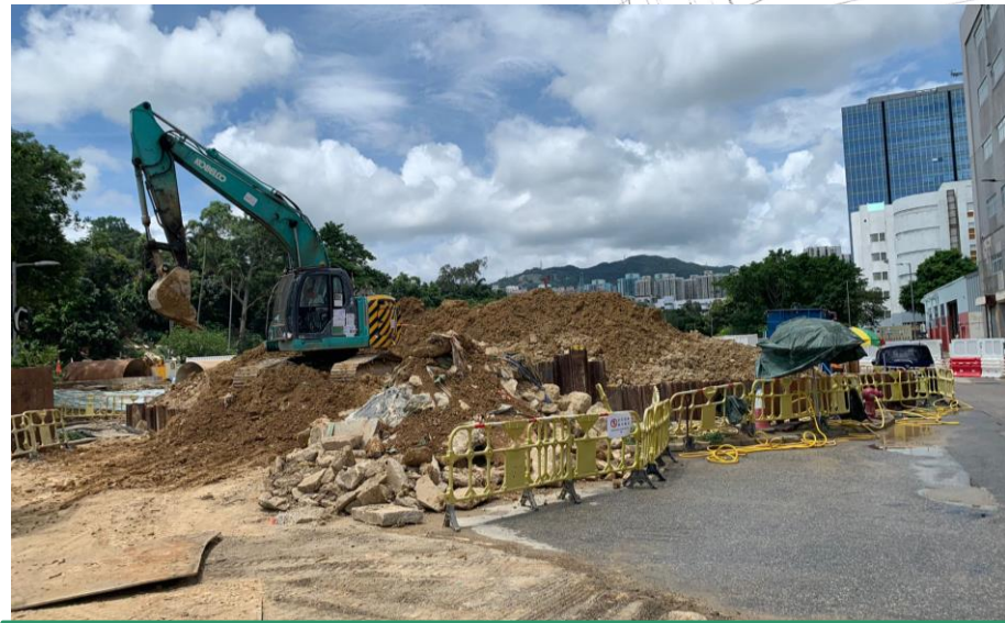
Wet Soil Storage and Treatment in C1-03
