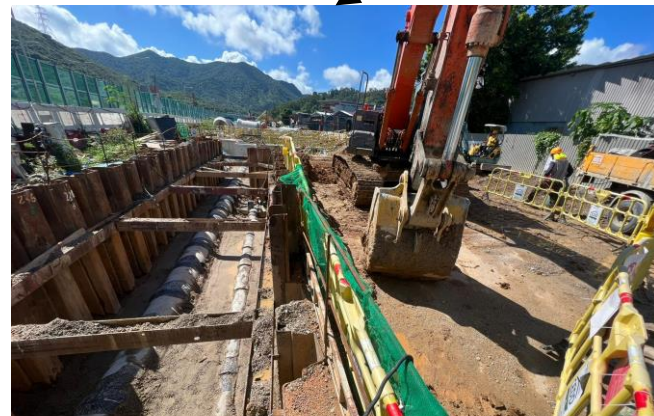
Dn600 Storm & Dn 450 Sewer
