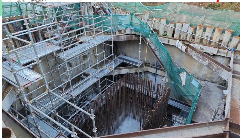
Concreting for C4-02 kicker for column completed on 06/07/22.
