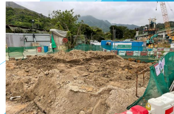
E1-04 Wet Soil Storage & Treatment
