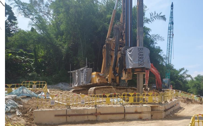
C2-03-P6 Bored pile in progress
