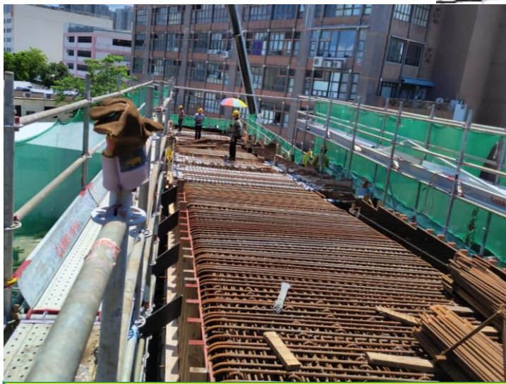
Rebar Fixing for C4-01 Portal Beam Construction (2 nd pour) in progress.
