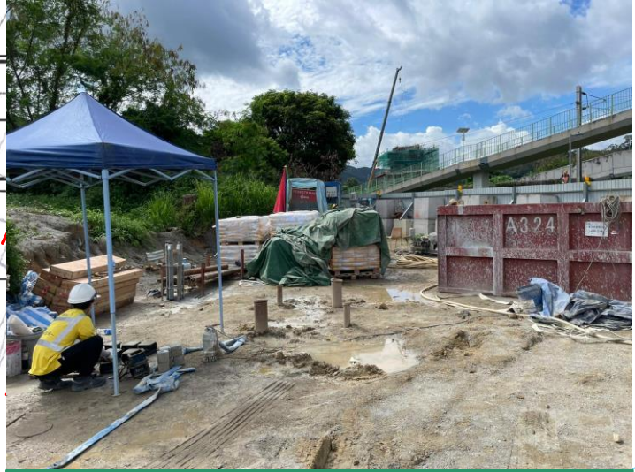
E2-01 bored pile reservation tubes grouting completed on 22/06/2022.
