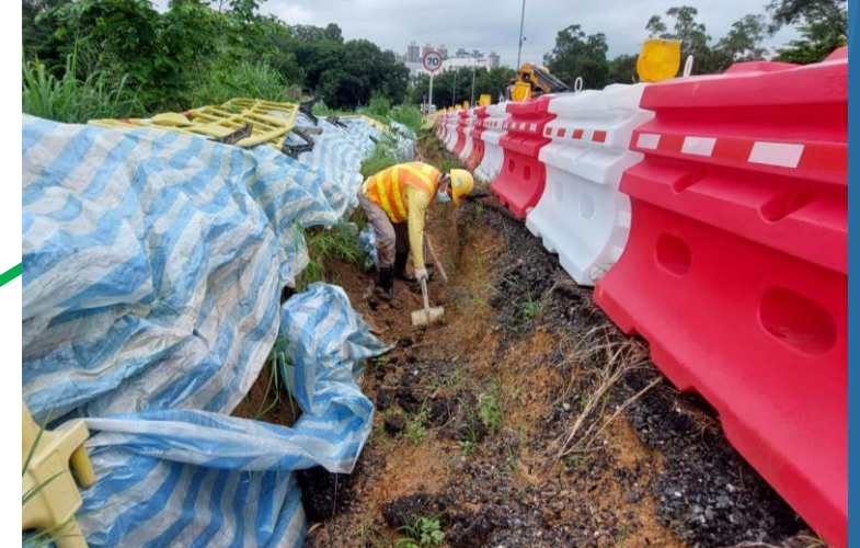
Excavate & Relocate CLP on Top of slope 3SW-C/F63
