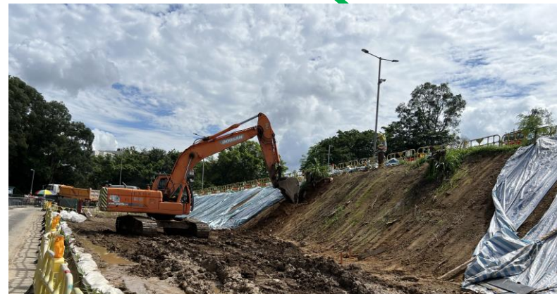
Removal of tree trunk and soil disposal for cut slope formation
