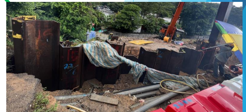
Sheet pile installation Sheetpiling works up to 05/07/22 Design review in progress for adoption of pipe piling to overcome underground obstruction
