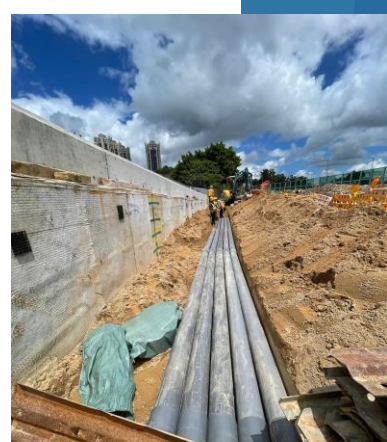
CLP 132 & 11kv ducting
