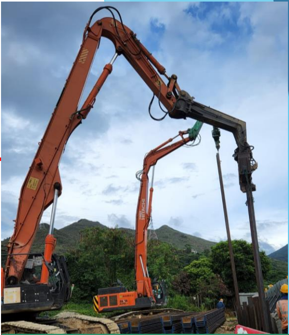
E2-01 sheet piling commenced on 28/06/22
