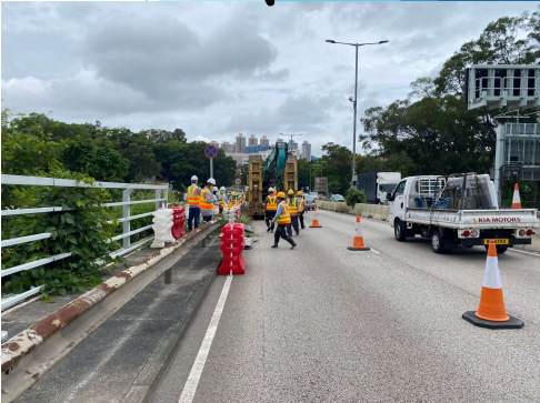
Sheet pile installation Slope works - ES:20/1/22- EF:6/5/22 - Slippage against R9
