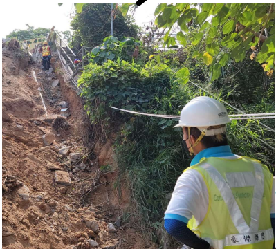
Breaking of existing step channel to facilitate the installation of sheet pile
