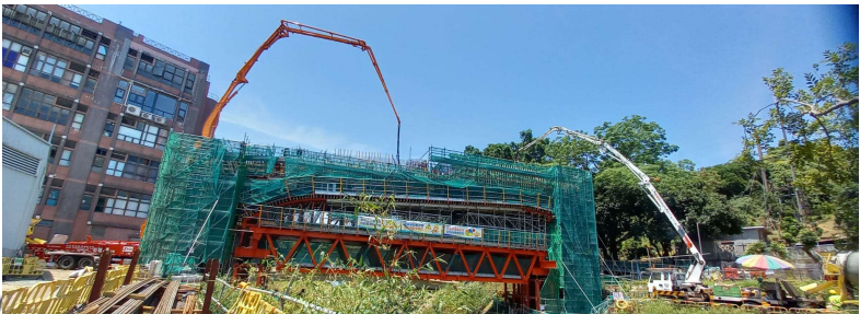
Concreting at C4-01 Portal Beam Construction (1 st pour) completed on 4-May-2022
