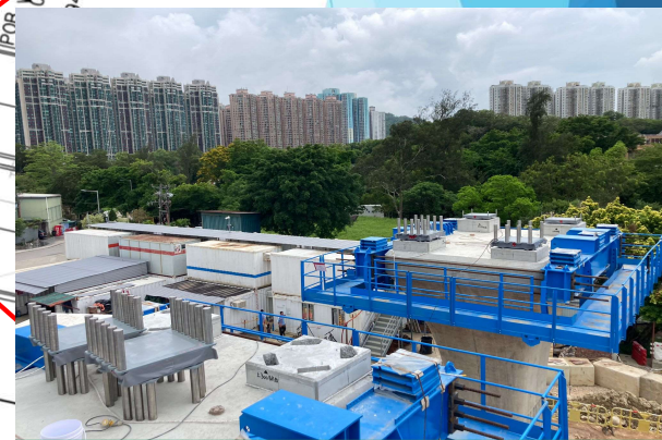
C4-04 aM & bM bearing plinths completed
