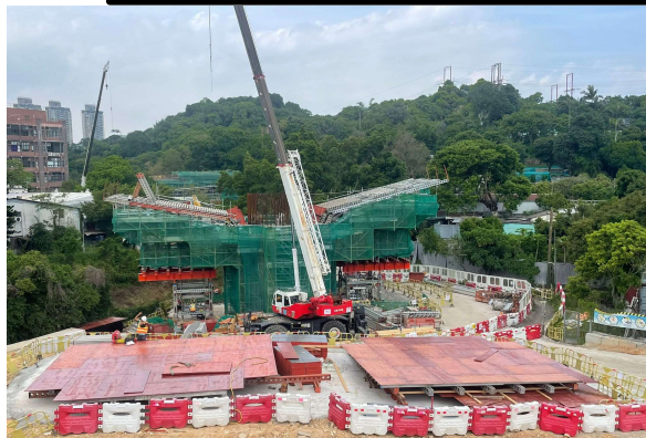
Falsework erection in progress for C4-03 Cross Head Construction.
