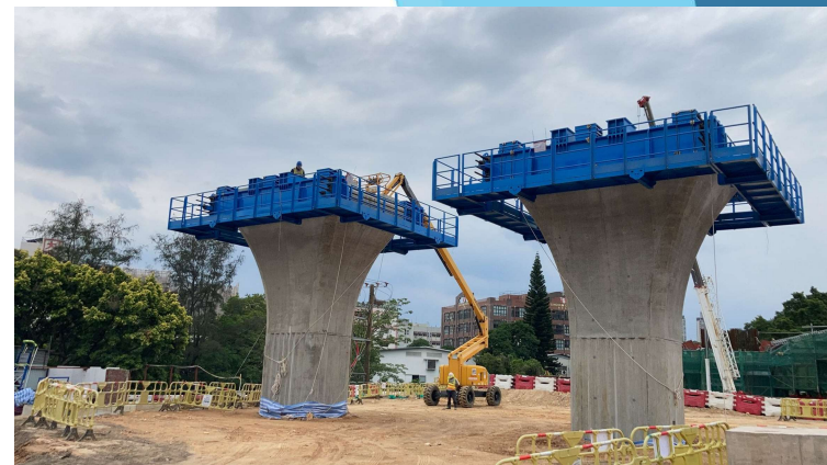
C4-04aM & bM Pier Head construction completed & hand over to bridge team on 26 Apr 2022
