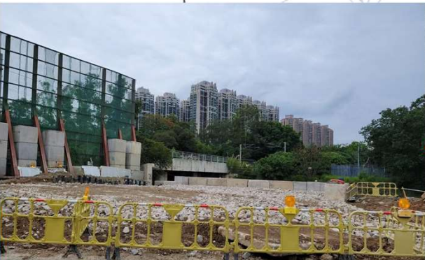
Concrete block piling platform completed on 7 May 22
