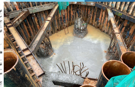
D1-04 Pile cap construction in Progress
