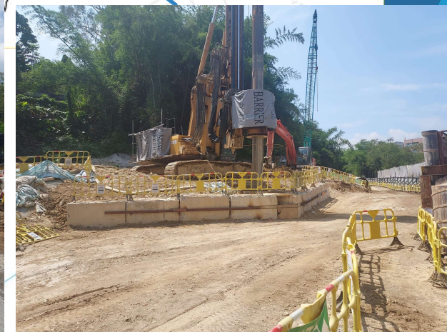
C2-03-P4 Bored pile in progress
