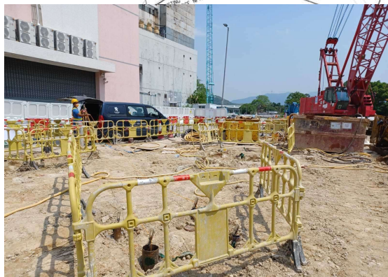
Bored Piles Testing works in C1-03
