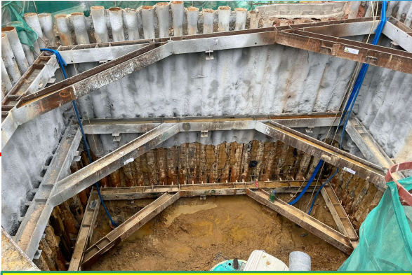
3 rd layer of waling & strut for C4-02 ELS is completed on 7/5/22
