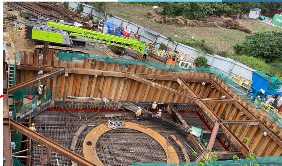
E2-01 lower pile cap rebar fixing in progress. Target to cast on 14/11/2022.
