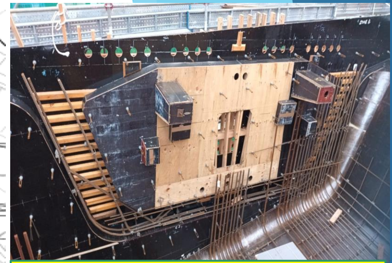
Rebar fixing for C4-02 cross head in progress
