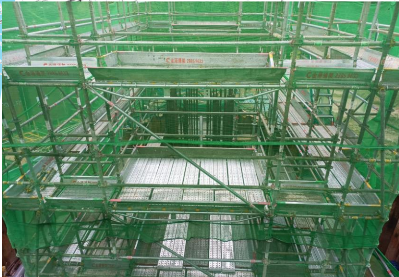
C1-03a pier head construction in progress
