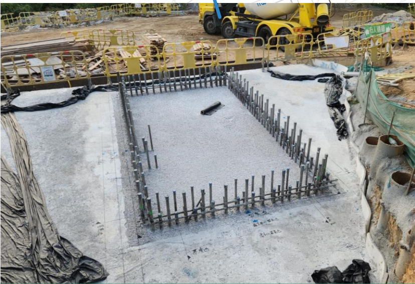
C3-01a pile cap completed on 27/10/22.
