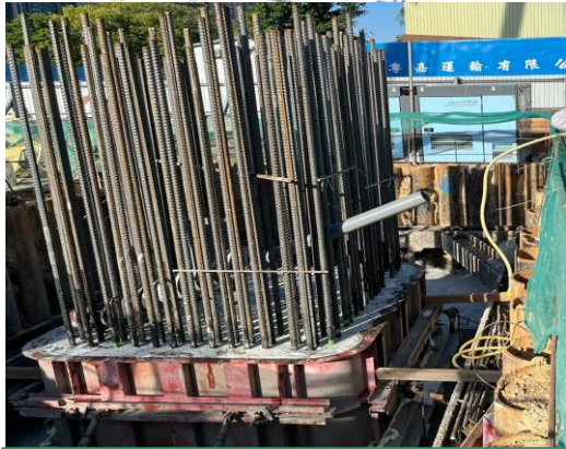
D1-02 pier (1 st pour) completed on 20/10/22
