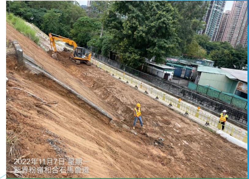
F63 Slope excavation for Ch. 50 - 110 Completed
