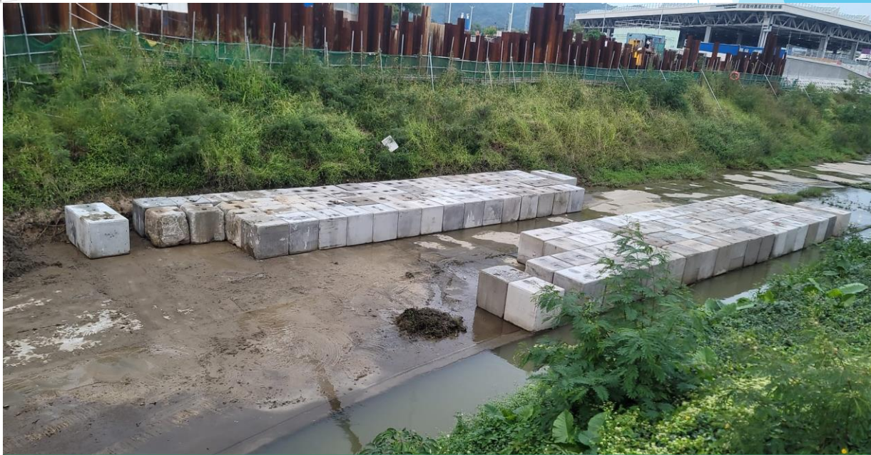
Construct concrete footing for B1-02 Portal falsework in progress.
