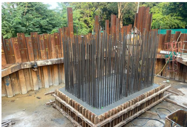
C2-02 kicker concreted on 09/11/22.
