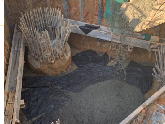
C2-03a cast blinding layer on 21/10/22.
