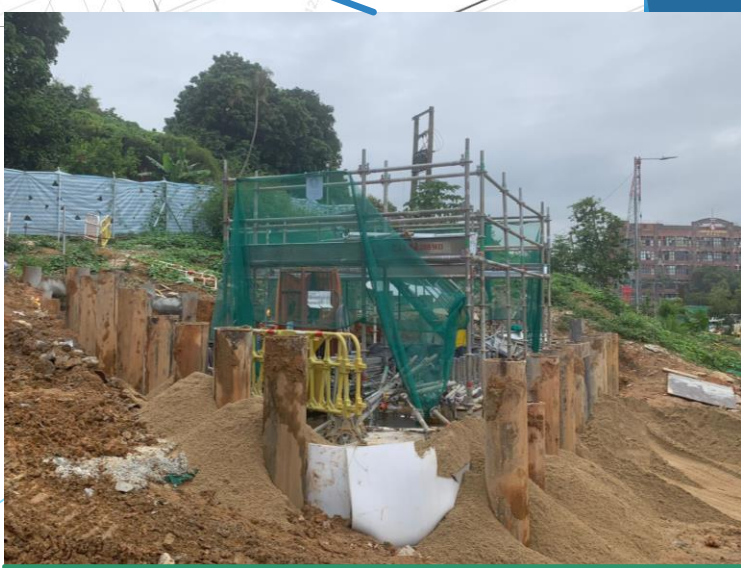
C3-01a pile extraction in progress.
