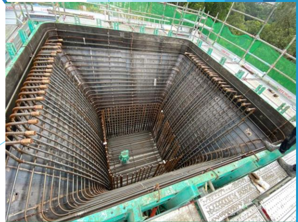
E1-04 pier head construction in progress
