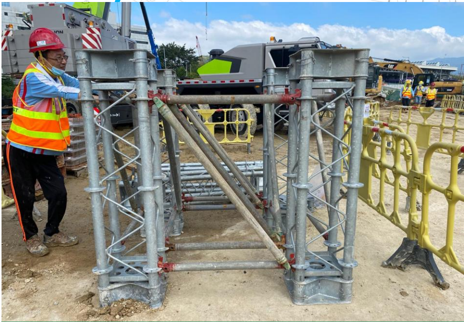
Erect RMD's Tetrashor for B1-02 Portal construction in progress.
