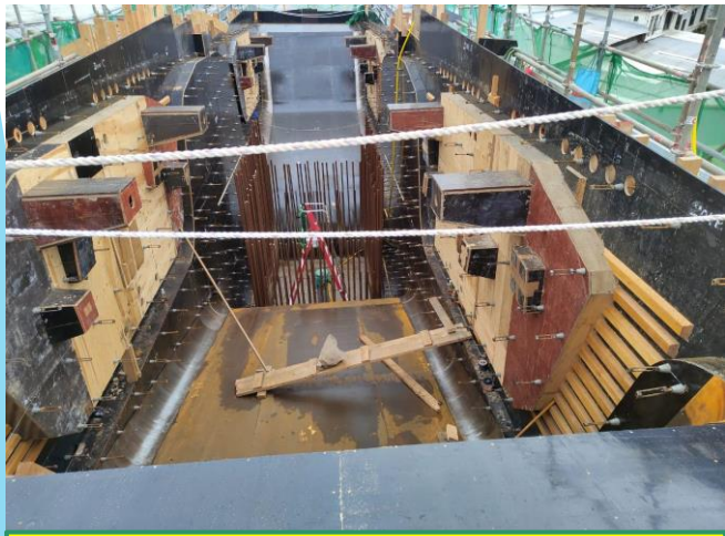
Formwork erection for C4-02 cross head completed on 05/11/2022
