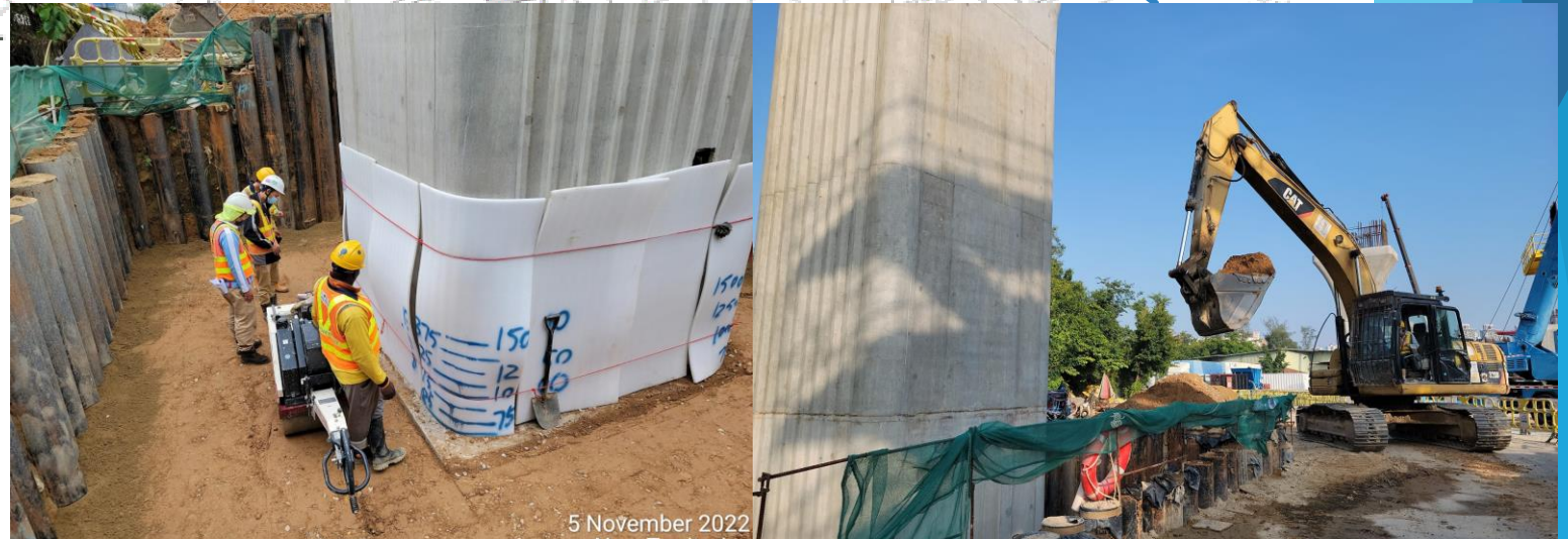
D1-04 backfilling in progress.
