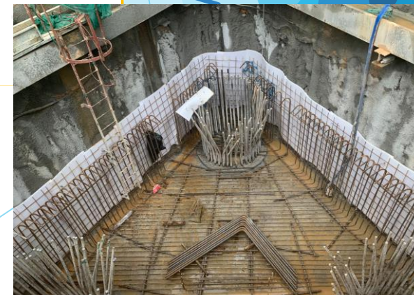
C2-03a pile cap rebar fixing in progress. Target to cast pile cap on 12/11/22.
