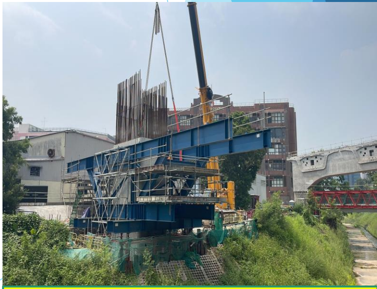
Temporary support beam platform C4-02 cross head construction completed on 04/10/22
