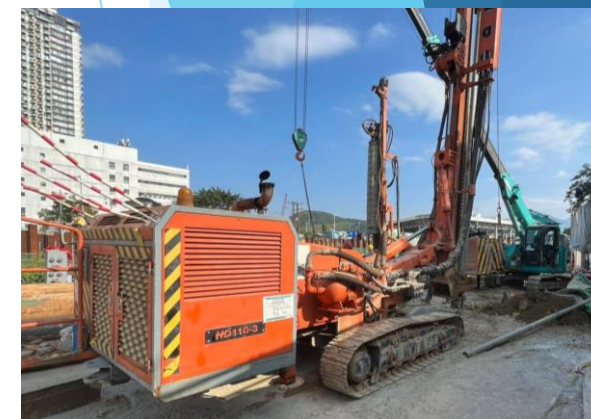
Portion II - B1-02a Pipe Piling Works in Progress
