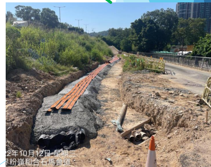
Concreting of CLP ducts completed on 11/10/22
