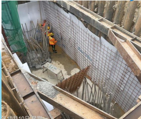
D1-02 blinding completed on 22/09/22. Rebar fixing commenced on 11/10/22.
