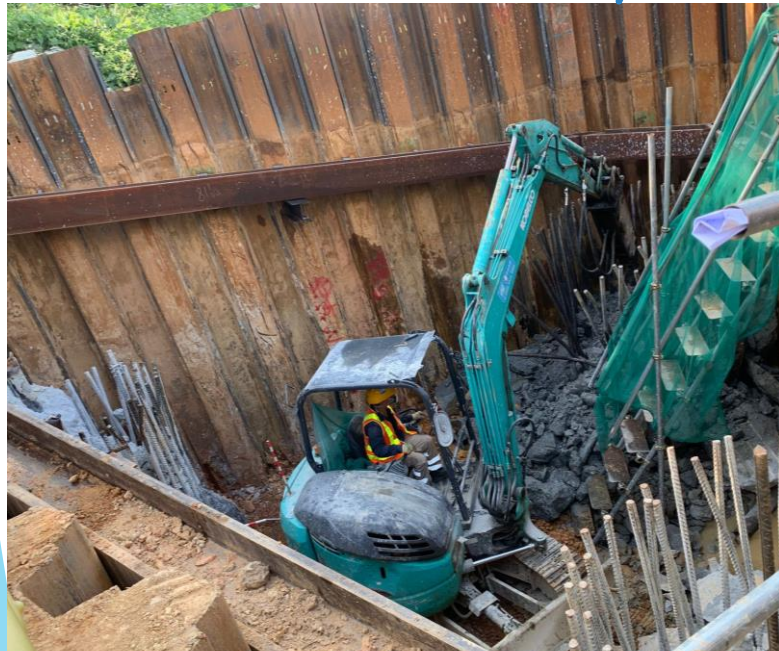
C2-04a sheet piling completed on 20/09/22, excavation and pile head breaking in progress. 1 st ELS layer completed on 30/09/22
