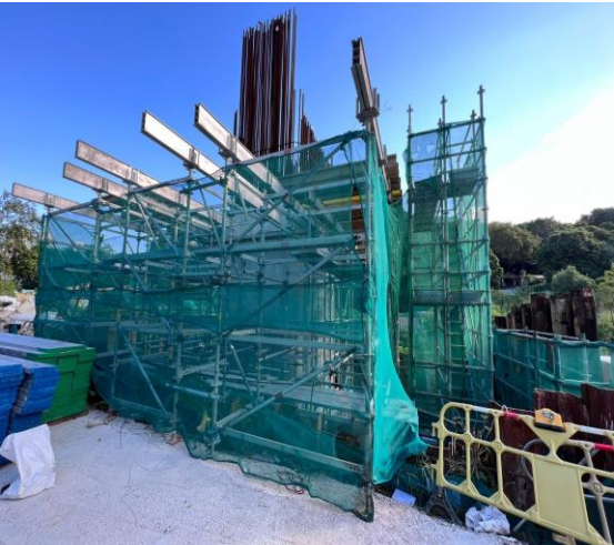
VST Tower at C3-03ab portal beam in progress
