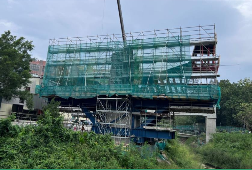
Formwork erection for C4-02 cross head soffit in progress
