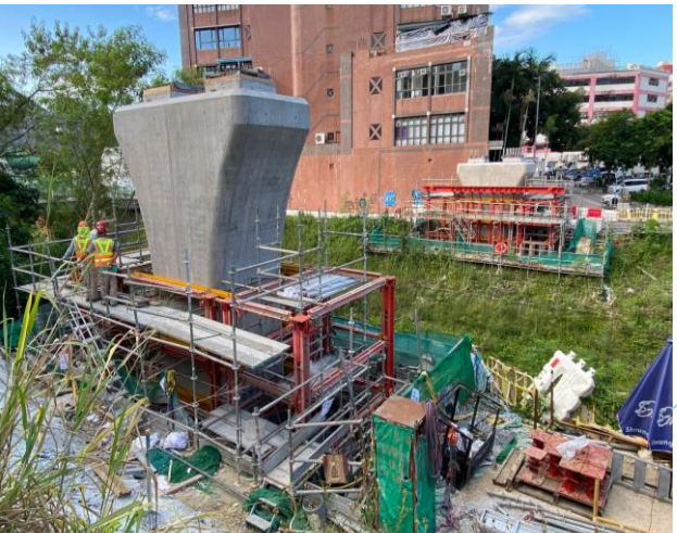
C3-04a pier head construction completed on 23/09/2022
