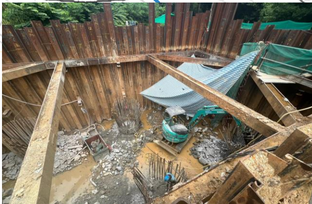
C2-02 blinding layer completed on 19/09/22. Breaking pile head in progress.
