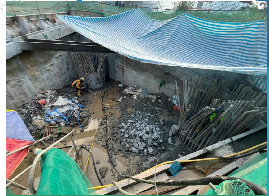
C3-01a pile head breaking in progress.
