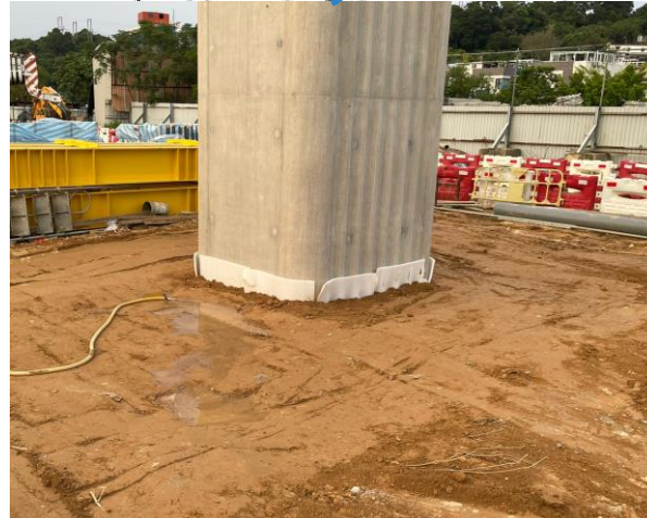
E1-03 backfilling to ground level and pipe pile extraction completed on 21/09/22
