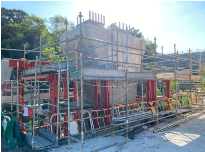
VST Tower at C3-04b portal beam completed on 8/10/22
