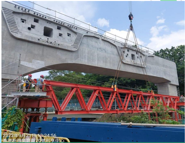
Dismantling of truss at C4-01 portal beam completed on 21/09/22
