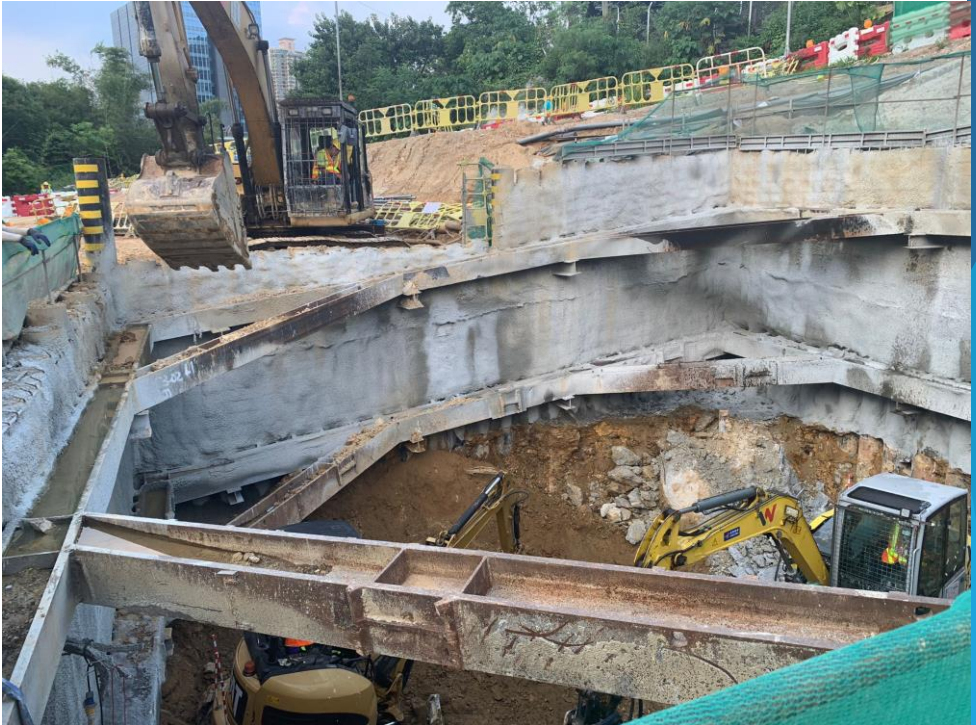
C3-02 Excavation to 3rd layer and rock breaking in progress.
