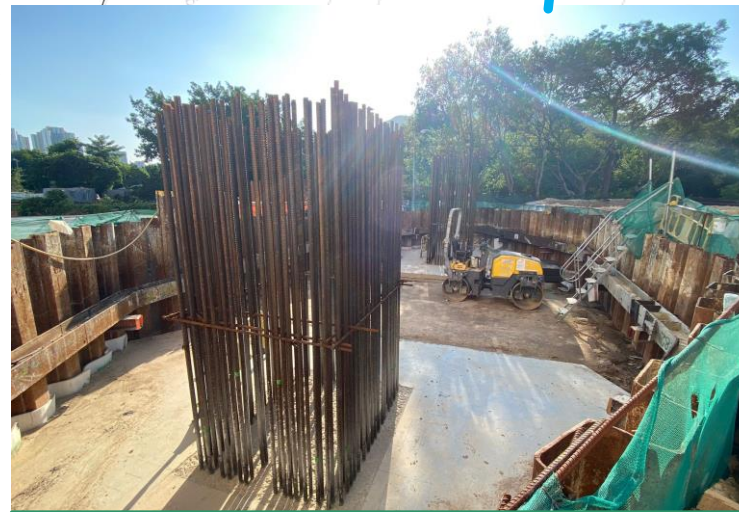
C1-03 backfill to pile cap top level completed on 11/10/22
