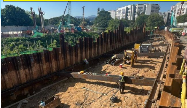
Portion 1 - B1-01M 1 st Layer Wailing/Struts Installation in Progress
