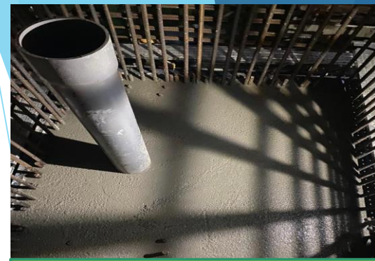
E1-04 pier (1 st pour) completed on 12/10/22
