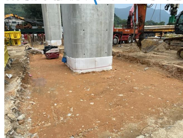
D1-03 backfilling to ground level and pipe pile extraction completed on 19/09/22
