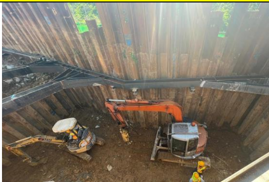
Portion 1 - B1-02b 2 nd Layer Wailing/Struts Installation in Progress
