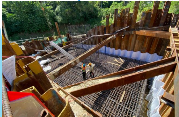
C2-01 blinding layer completed on 13/09/22. Rebar fixing in progress.
