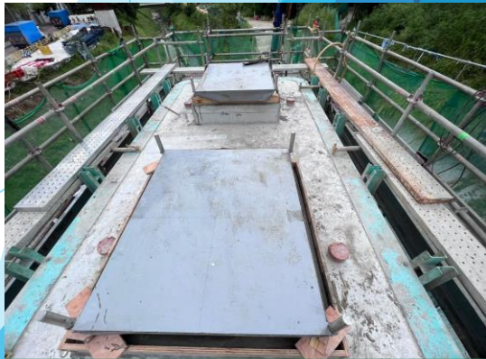
C3-04a bearing plinth completed on 24/09/22
