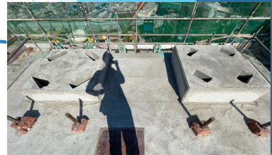
D1-04 Bearing plinth completed on 11/10/22
