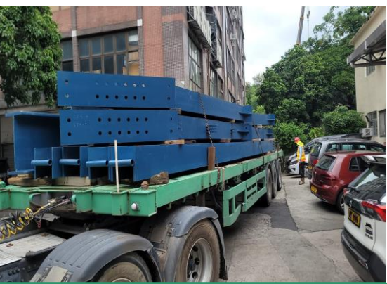
Support H beam for C4-02 cross head construction arrived on site on 7/9/22
