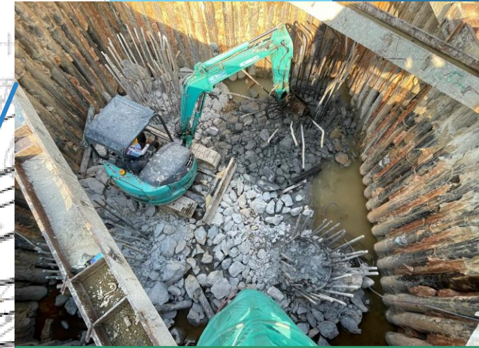
E1-04 pile head breaking in progress
