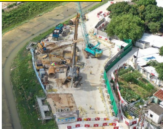
Portion II - Bored Piling Works in Progress
