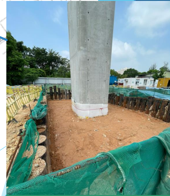
D1-03 backfilling to ground level in progress
