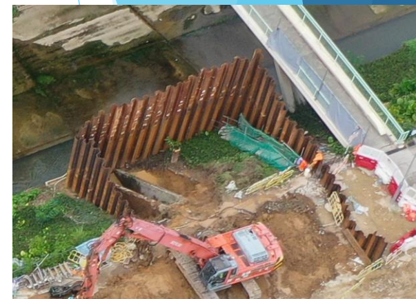
Portion II - Demolition of River Gauge Wing Wall completed
