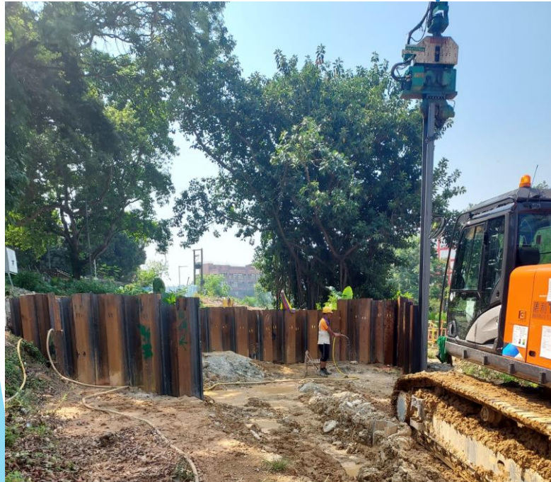
C2-04a Sheet Piling commenced on 31/08/22
