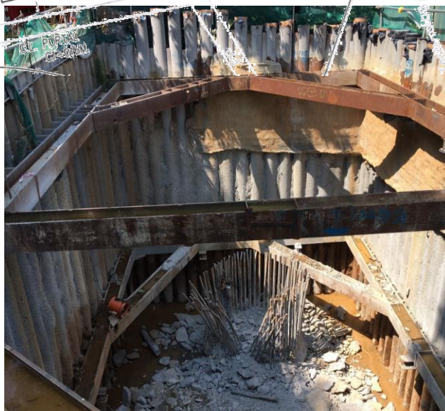
C1-01b Sprayed Concrete for Pipe Pile wall and Concreting of blinding layer completed on 26/08/22
