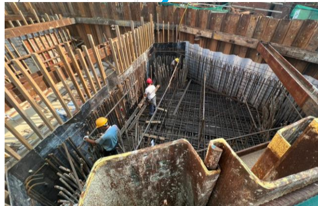
Rebar fixing for C1-03a pile cap in progress
