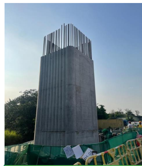
D1-04 Pier Construction completed
