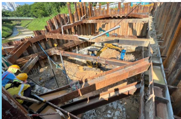
C2-01 2 nd layer strut completed on 01/09/22. Excavation to founding level in progress.
