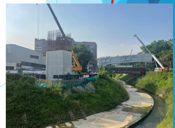
C4-02 cross head construction in progress.
