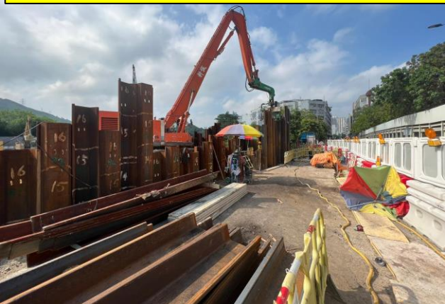
Portion 1 - Sheet Piling works for Abutment B1 & Cap B1-02b in progress
