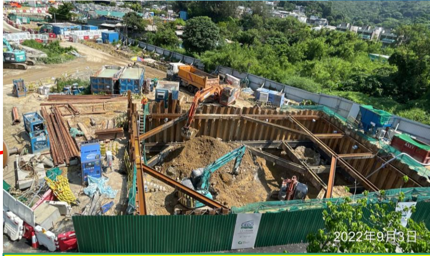
2nd layer strut completed on 31/08/22. Excavation to 3rd layer strut in progress.
