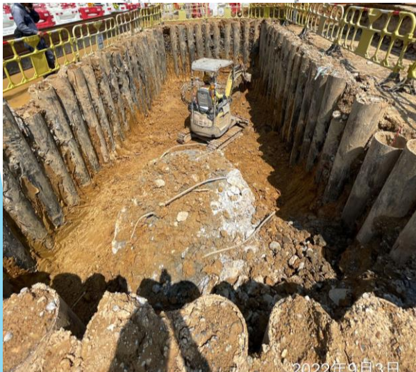
Pipe piling for D1-02 completed on 31/08/22
