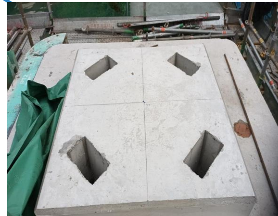
C3-04b Bearing Plinth completed on 07/09/22
