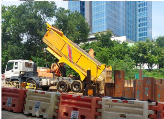
Temporary wet soil storage in C2-02 cofferdam
