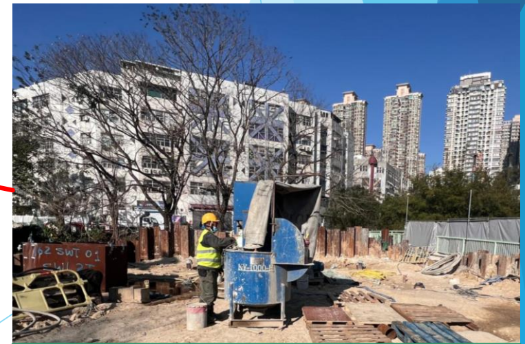
B2-03 Grouting of reservation tubes Completed
