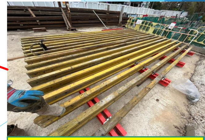
C1-01b pier head construction in progress
