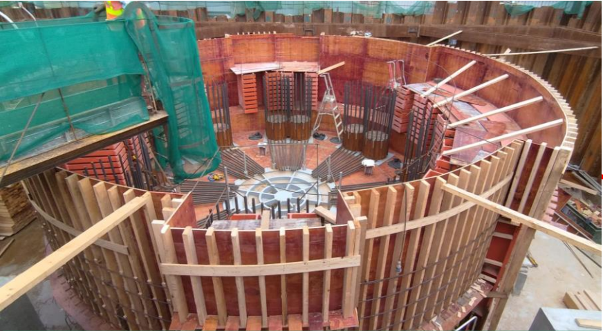
E2-01 formwork erection for upper turntable in progress.
