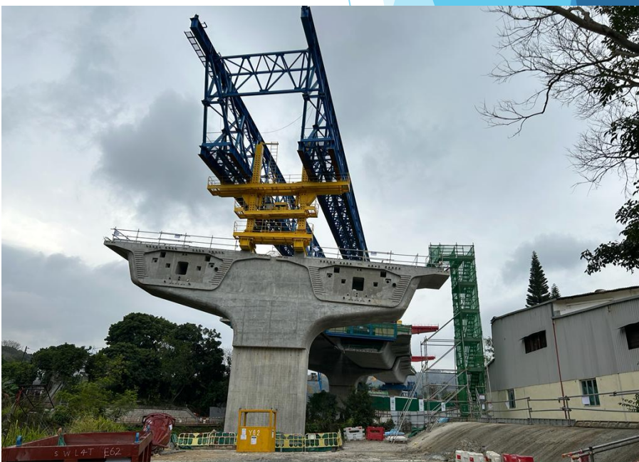
C4-02 Dismantling of temporary falsework completed on 13/01/23
