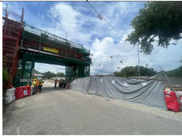
Provision of noise barrier for noisy works in Long Valley
