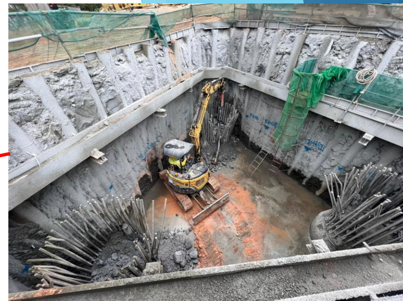
C3-01b blinding layer completed on 03/02/23. Pile head breaking in progress.
