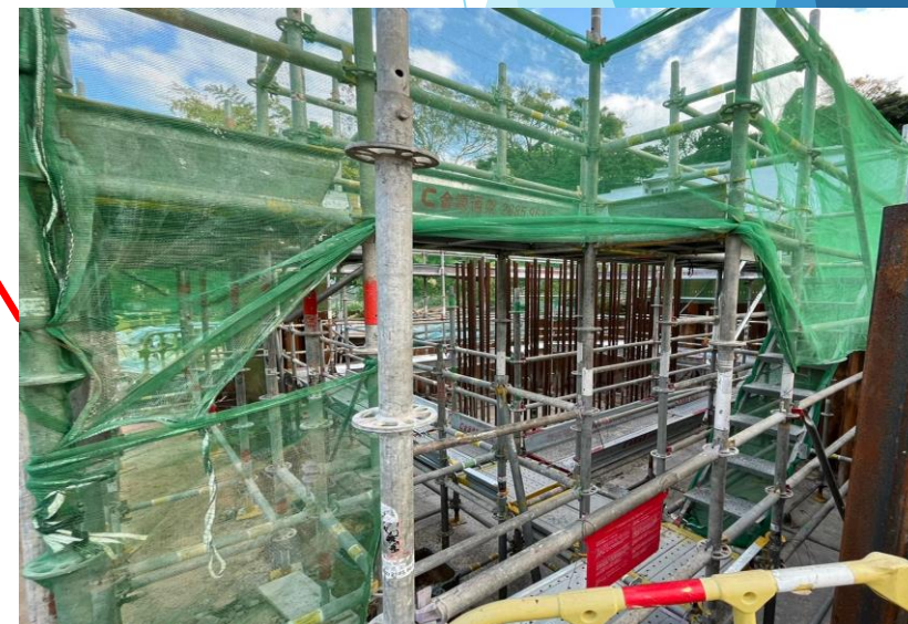
C2-04a pier head construction in progress
