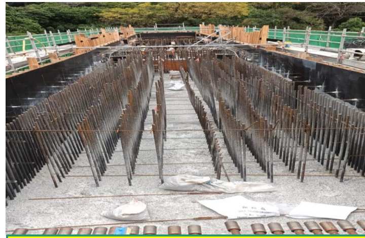
C3-03 Portal Beam rebar fixing for 2 nd pour in progress
