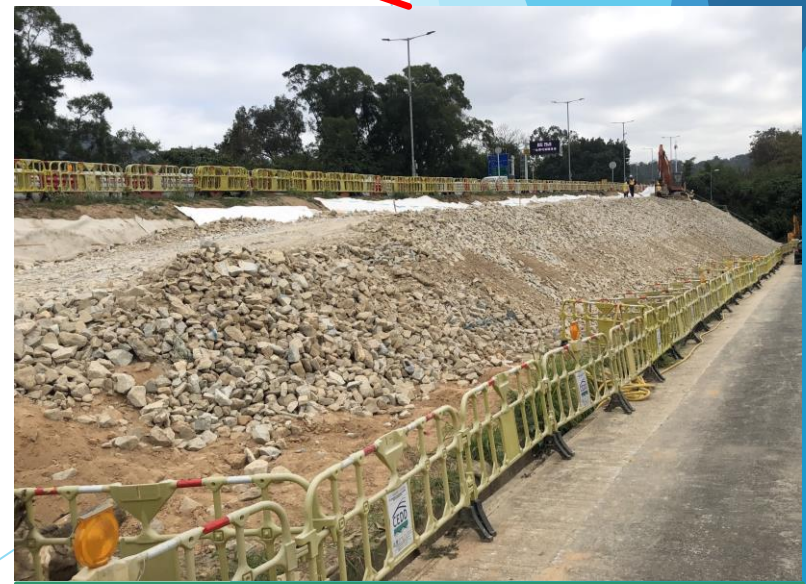
Rockfill Slope at Ch. 0 - 110 in progress
