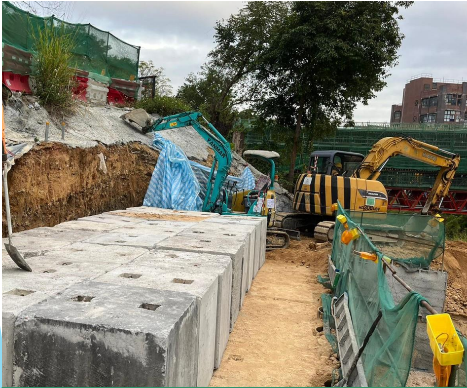
Footing for C3-02 cross head construction in progress
