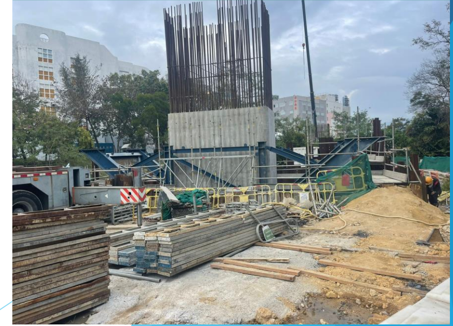
C2-02 cross head construction in progress
