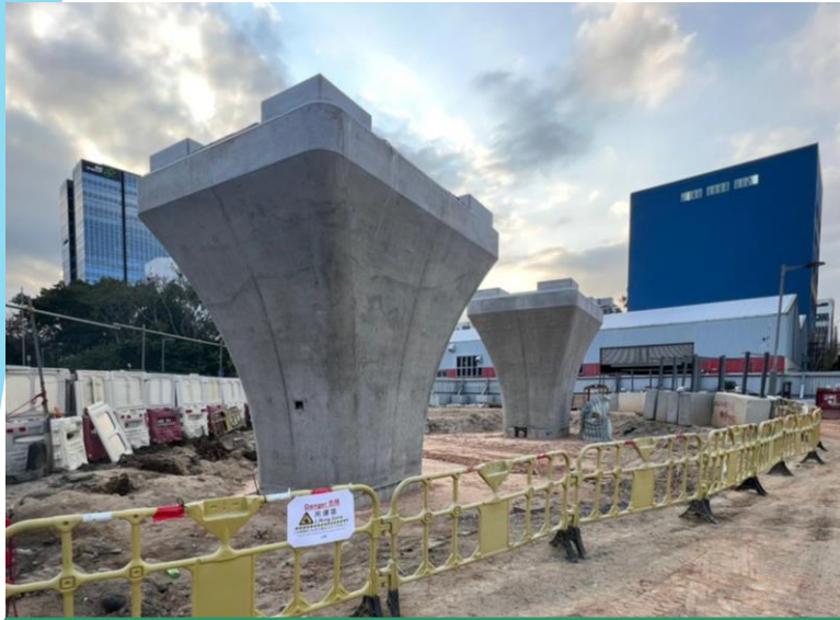
C1-04 sheet pile extraction completed on 06/02/23. Backfilling to E.G.L. in progress.
