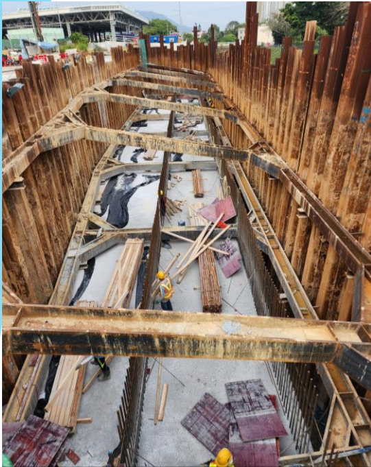
B1-01M Pile Cap Concreted & Formwork Removal works in progress
