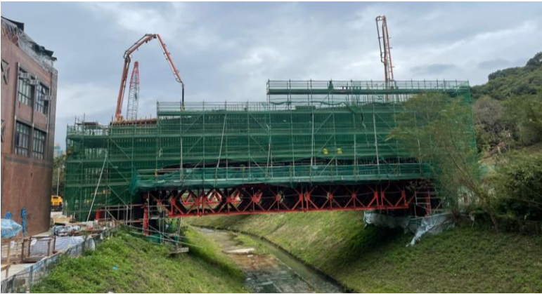
C3-04 Portal Beam 1 st pour concreting completed on 12/01/23
