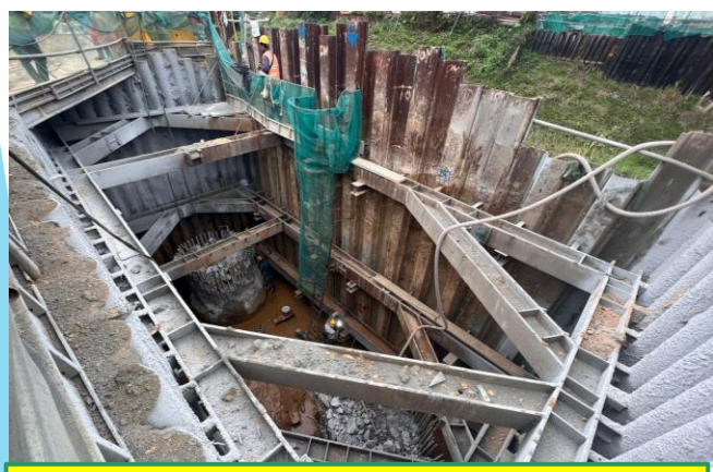
C1-01a 3rd layer of strut Installation completed
