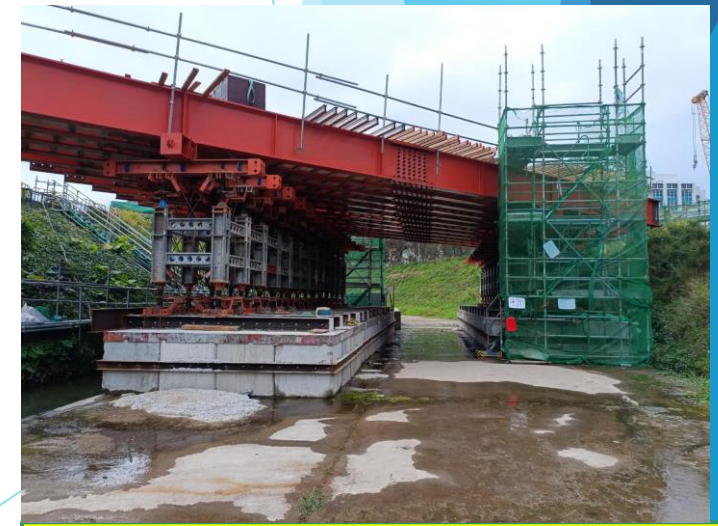
B1-02 Mega-shor tower for portal beam construction completed on 29/12/22
