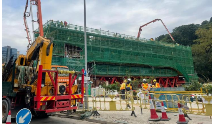
C3-03 Portal Beam 1 st pour concreting completed on 19/01/23
