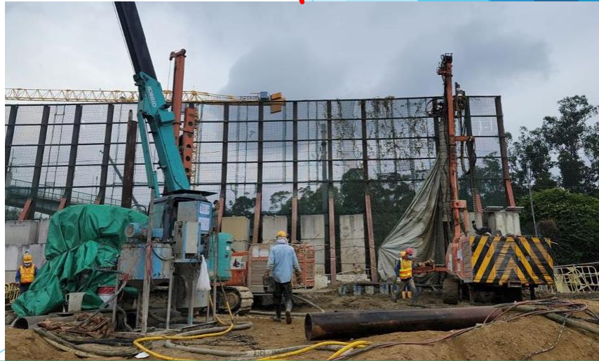
D2-01 pre-grouting works (within MTRC 6m Zone) completed. Pipe piling in progress.
