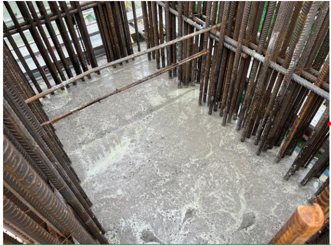
C1-02a pier 1 st & 2 nd pour completed on 20/01/23 & 03/02/23 respectively
