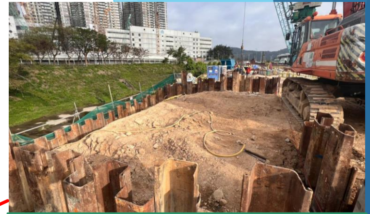
B2-02 Sheet Piling Works in progress
