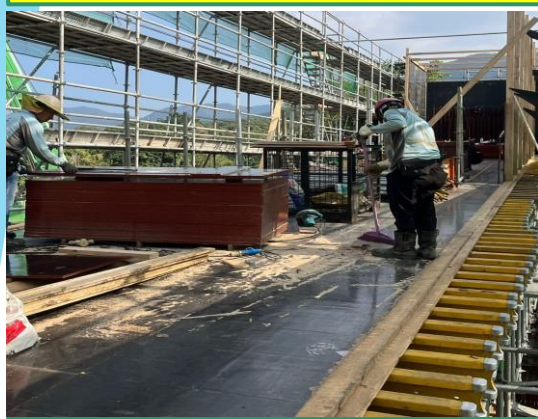
Soffit formwork for C1-02 portal beam construction completed 08/12/23
