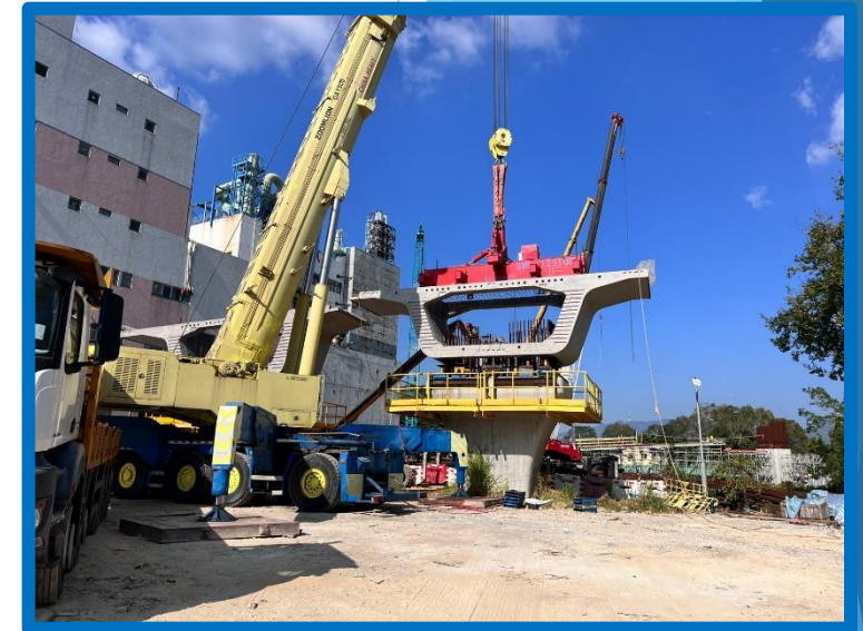
Precast cell at C1-03 erected on 14 Nov 2013
