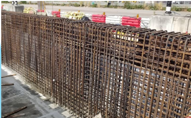
NB109 Bay 12 Wall - Rebar fixing completed
