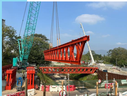
Truss erection at C1-01 MJ portal is progress
