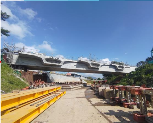
Dismantling of soffit & steel beam at B1-02 portal beam completed on 12/12/23.
