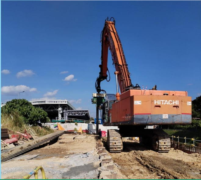
Sheet pile extraction (near C4) completed on 04/12/23
