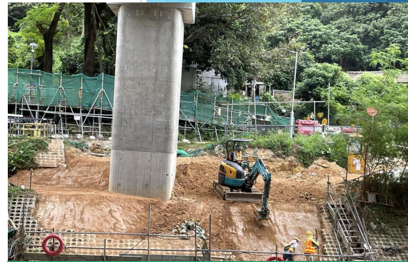
Trimming pipe pile and cut slope profile completed on 15/11/23
