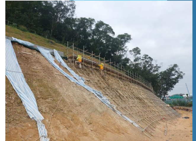
Erected working platform for berm and rock mapping
