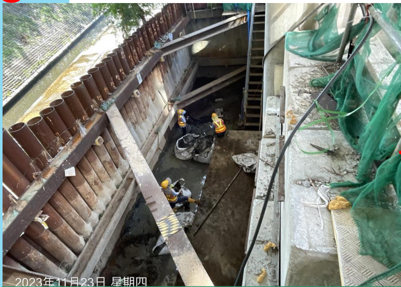
Site clearance at C4-01b cofferdam before backfilling
