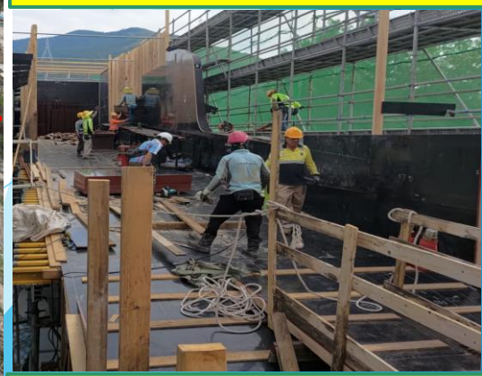
Side formwork erection at C1-02 portal in progress
