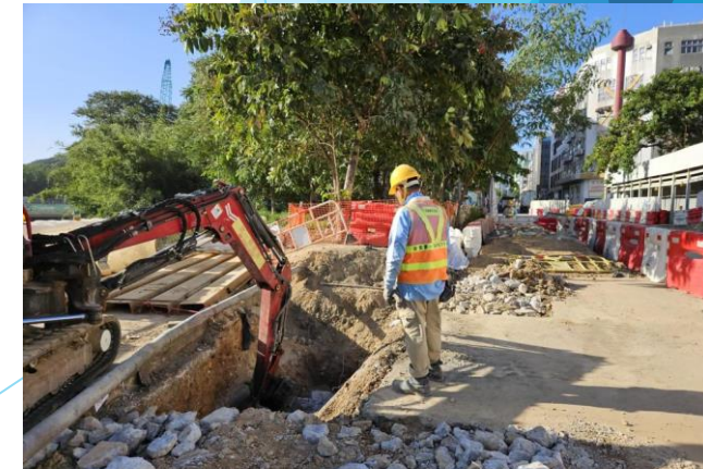
Excavation for Manhole SMH_FL8701 in progress.
