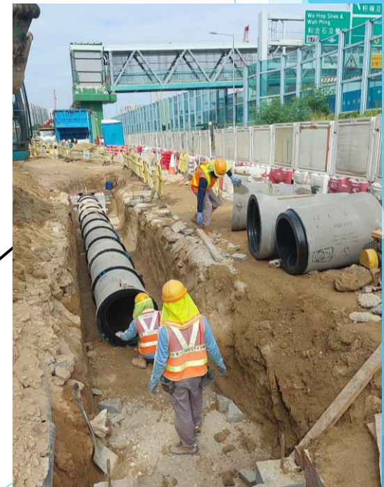
Laying DN600 Sewerage Pipe at FW06
