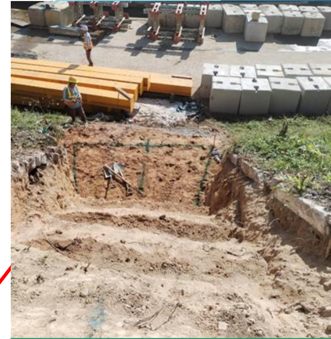
Excavation for DN900 and Outfall FL8701 in progress.
