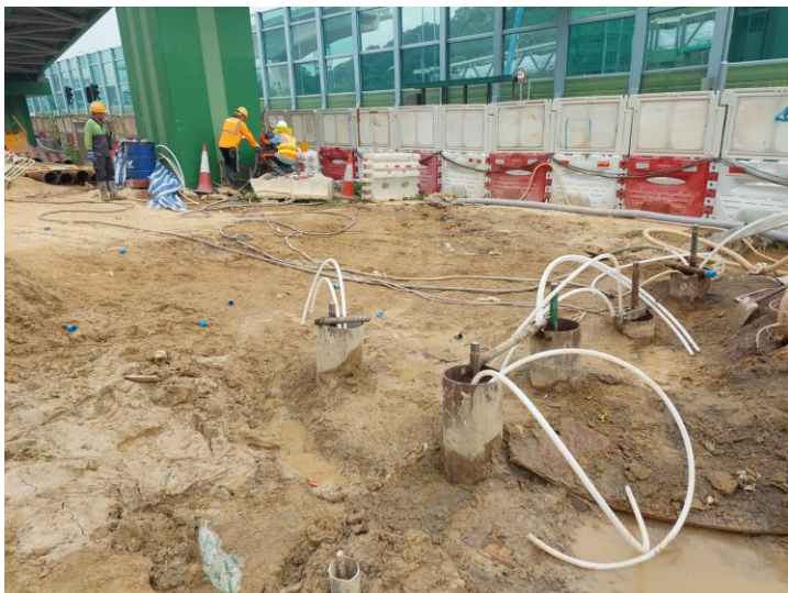
LT2 Piling Works in Progress (12 out of 19 Minipiles completed) Target Completion 23/12
