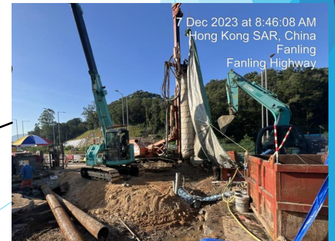
E4-02 Pipe pile wall in progress
