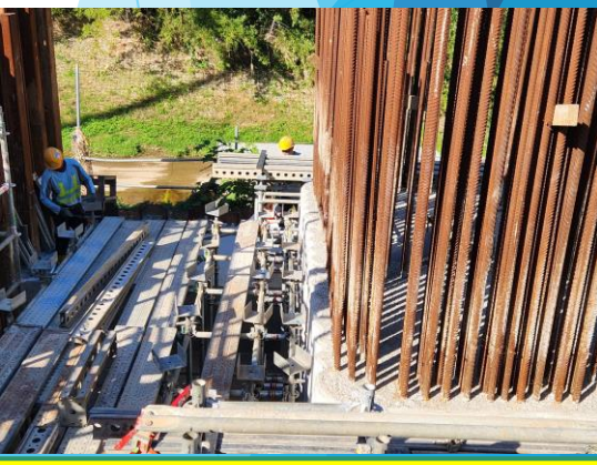
Falsework erection for B2-02 cross head construction in progress
