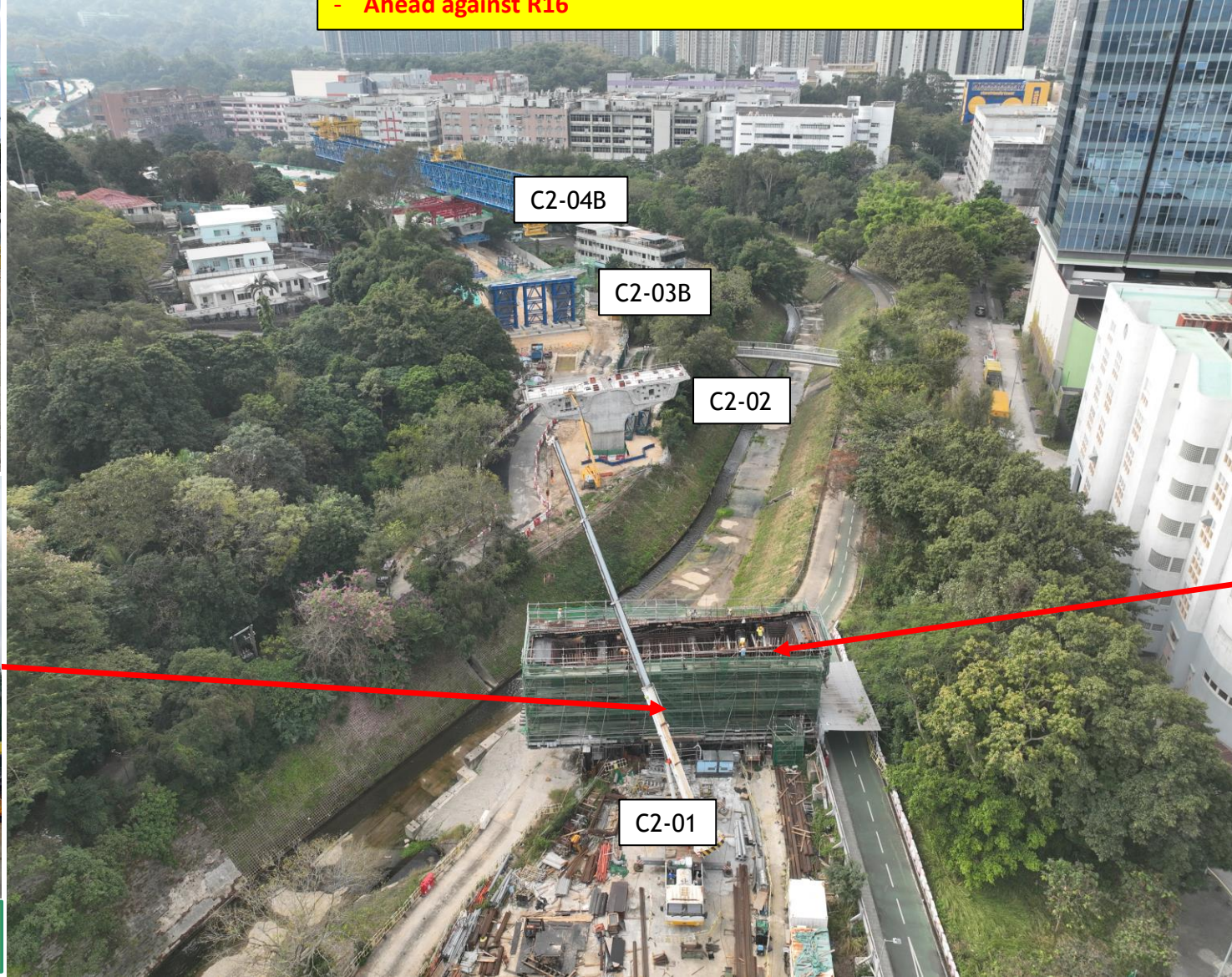
1 st Concreting for C2-01 cross head completed on 30/11/23
