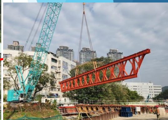
Truss erection at C1-01 MJ portal is progress
