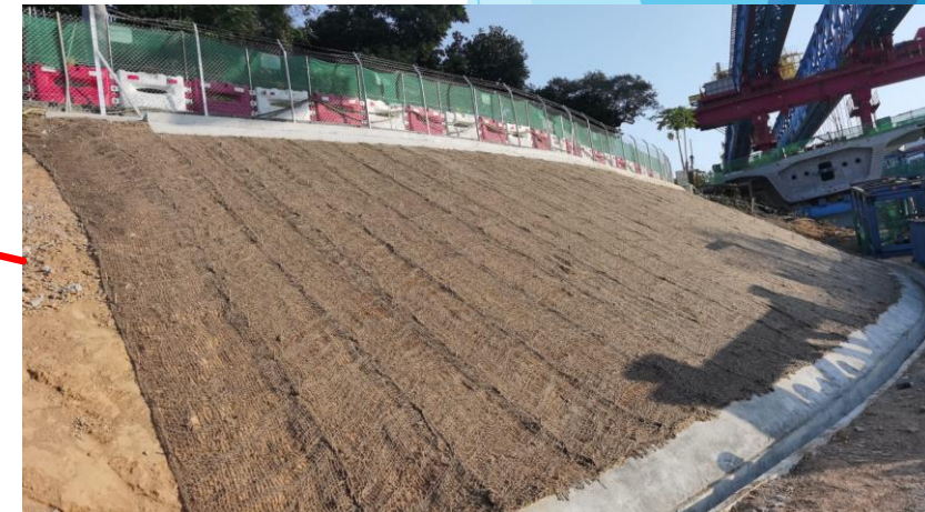
Laying erosion control mat at slope FS30 completed on 18/11/23
