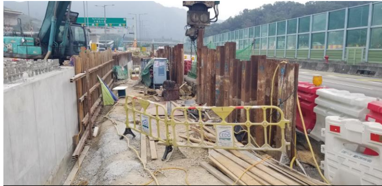
NB109 Bay 6-8 extracted remaining sheetpiles
