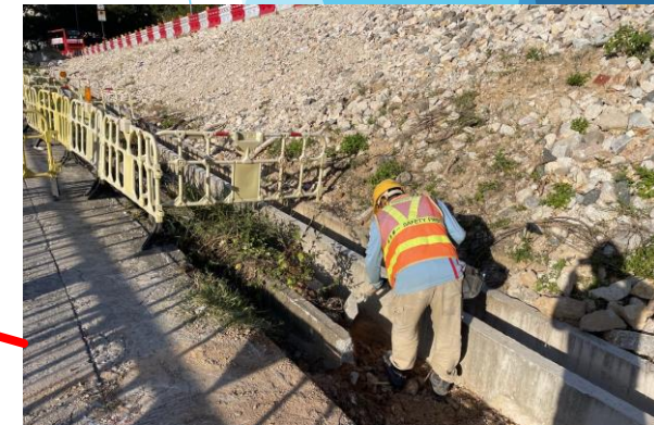
Excavation for WSD fresh watermain laying in progress.
