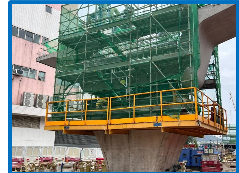
Construction the diaphragm of C1-03 in progress
