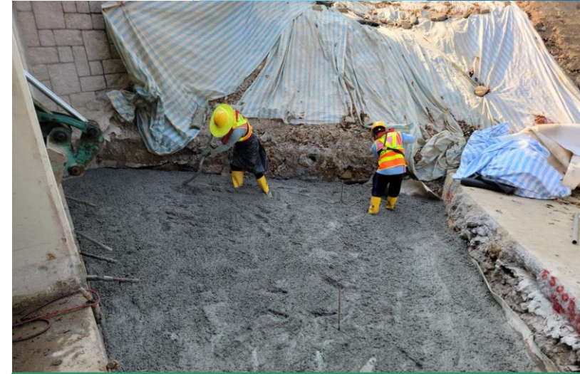
Casting of blinding layer for box culvert extension completed. (27/11/2023)
