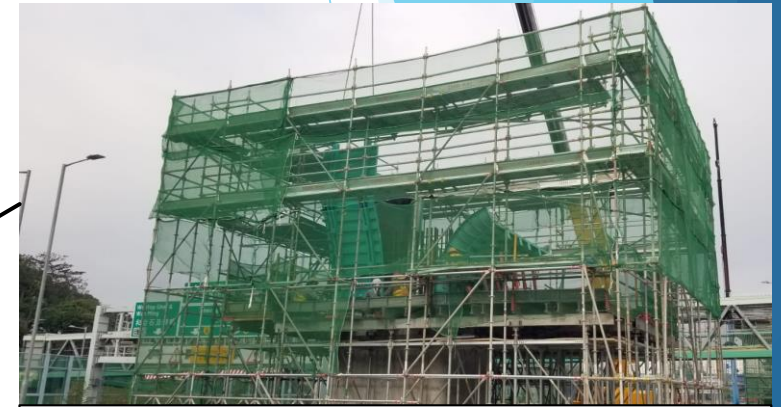
E3-05M Pierhead Steel Mould Erection in Progress
