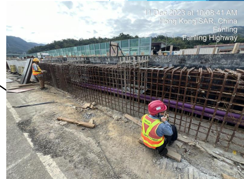
NB109 Bay 6,8 - Noise Barrier HDBs installed on 8/12
