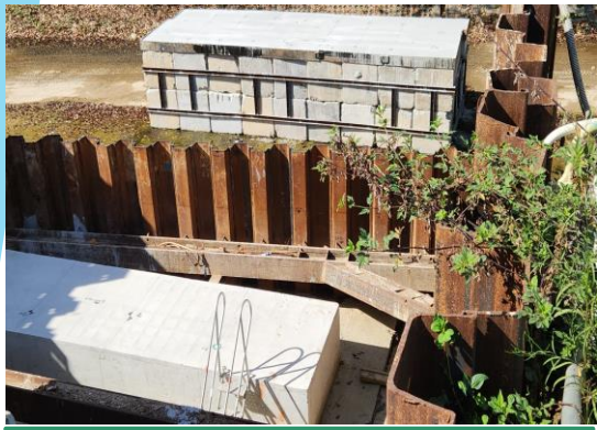
Mass concrete for B2-03 cross head construction completed.
