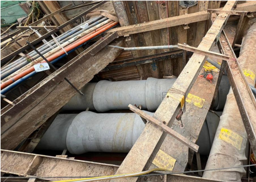
Installation of 2xD1200 Stormwater Pipe completed on 14/12
