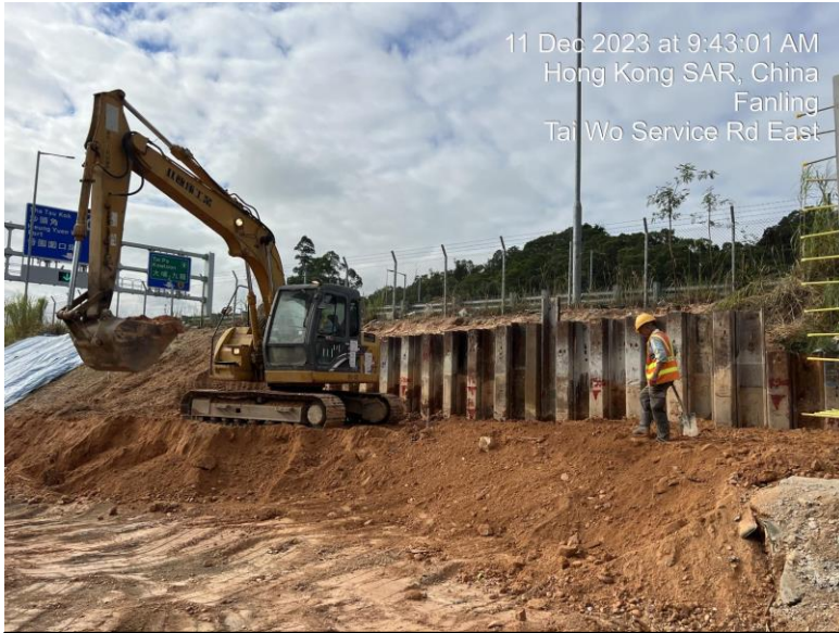
NB110 Bay 9 sheetpiling in Progress
