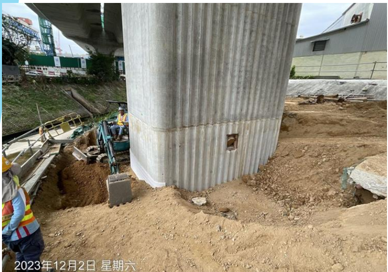
Backfilling at C4-02 ELS cofferdam in progress. SRT at +10.4mPD passed.
