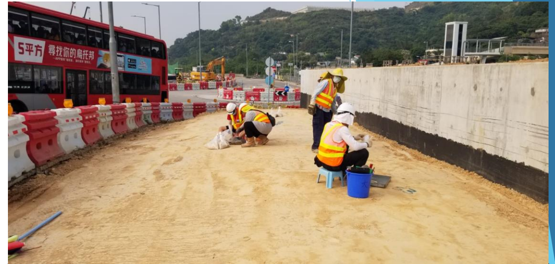
NB110 Bay 3-5 Backfilled to Formation
