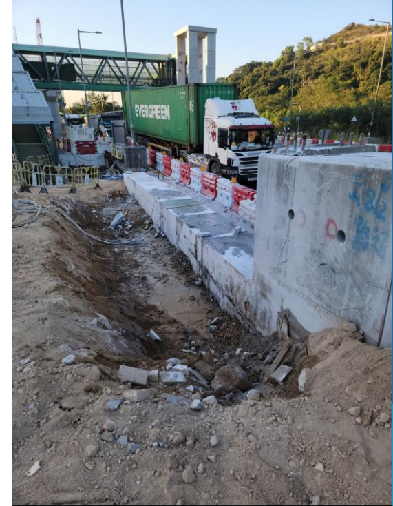
NB74 Stem wall removed by saw cut on 11/12.
