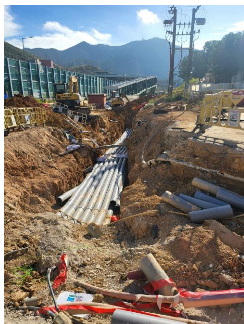
CLP laying ducting for 11kV
