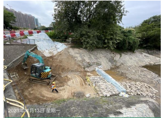
Excavation for box culvert extension & breaking of base slab completed.
