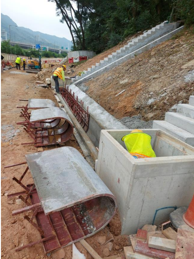
Casted 600UC between CP8 and CP9 CP10 is in progress
