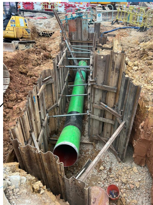
TownGas laying DN600 pipeline
