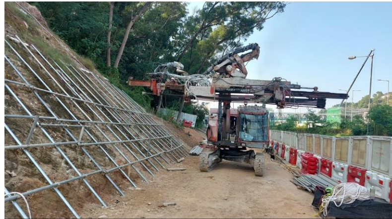
Remaining Raking Drain at FS04 completed
