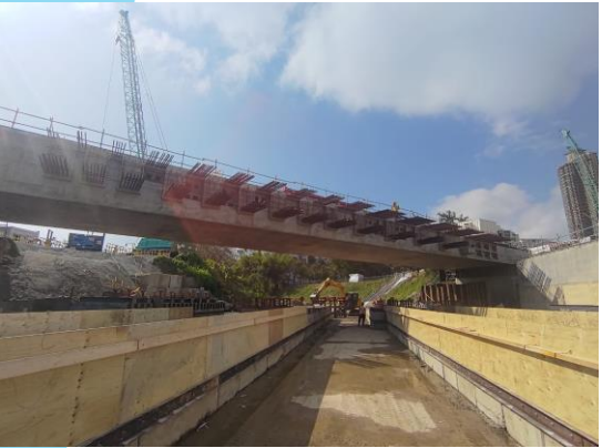
Dismantling of soffit & steel beam at B1-02 portal beam completed on 12/12/23.
