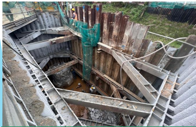
C1-01a 3rd layer of strut Installation completed
