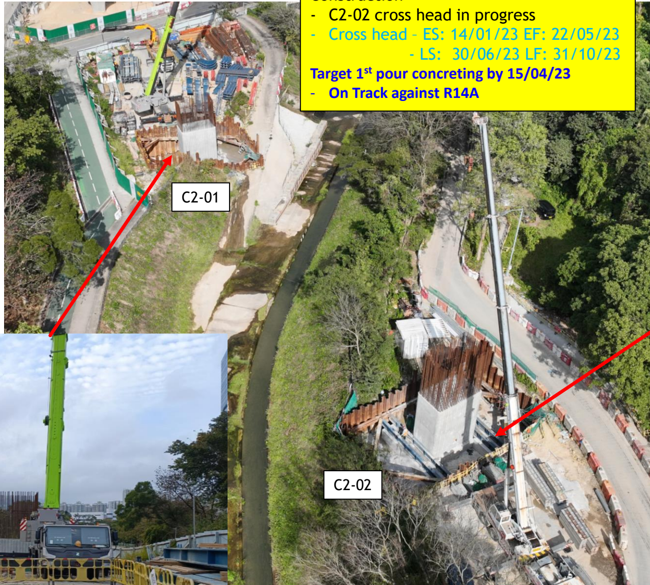
C2-01 Dismantling of falsework completed
