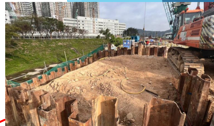
B2-02 Sheet Piling Works in progress
