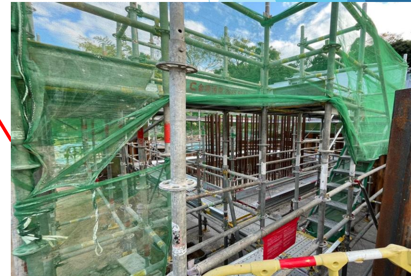
C2-04a pier head construction in progress
