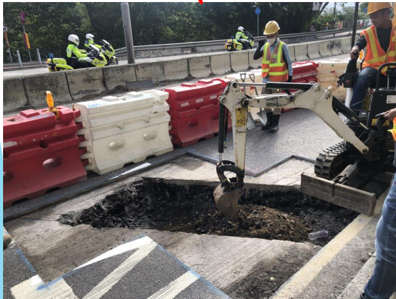
Trench excavation for watermain diversion (near FS05)
