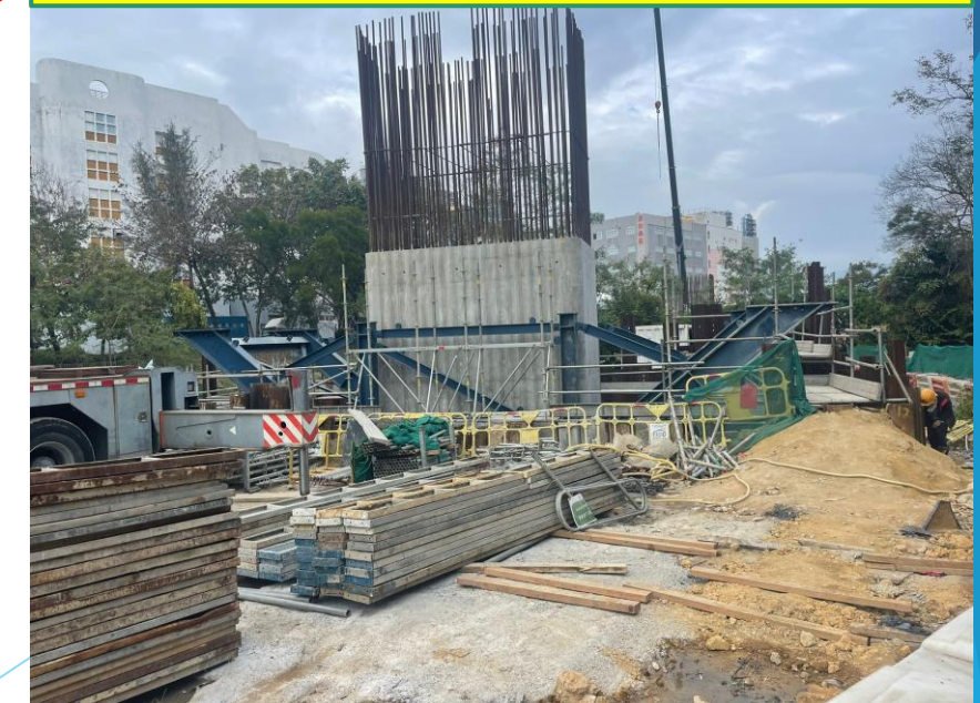
C2-02 cross head construction in progress
