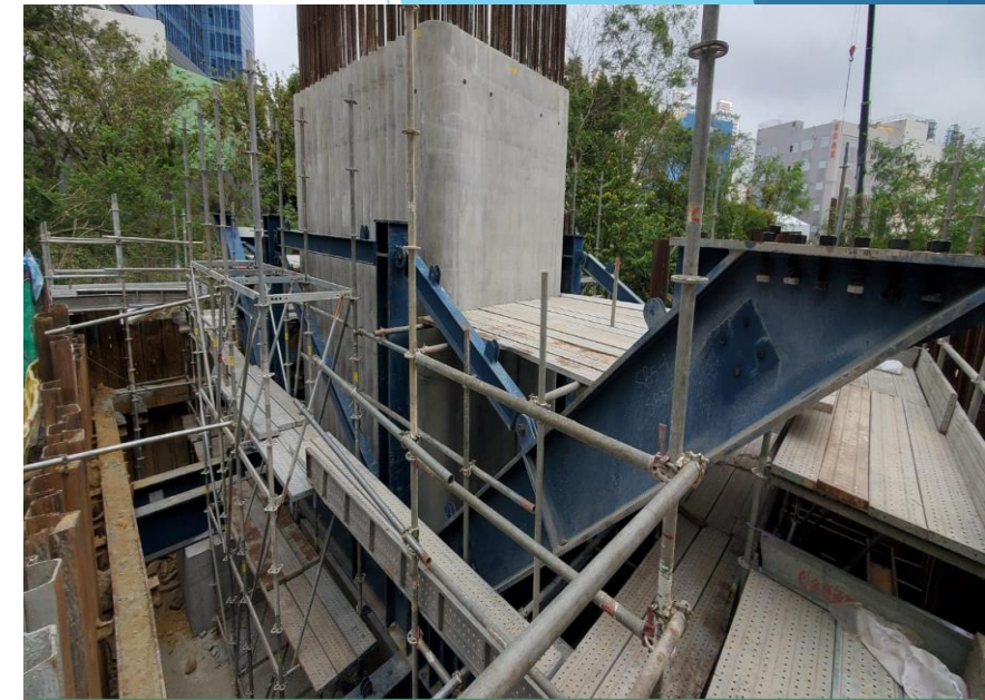
C2-02 cross head construction in progress
