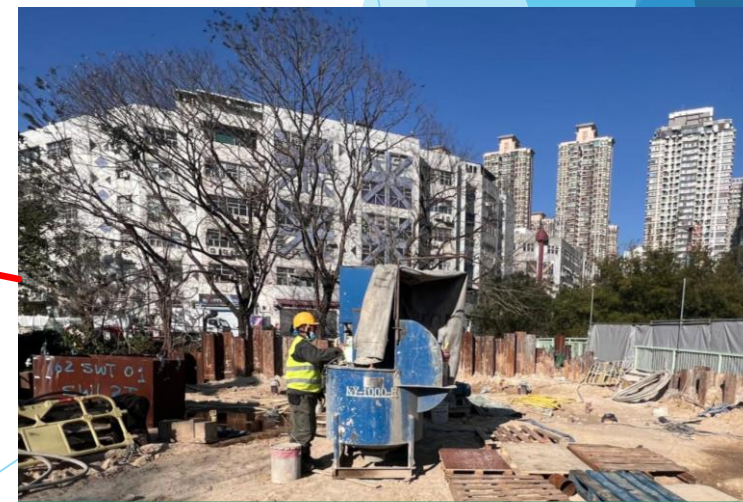
B2-03 Grouting of reservation tubes Completed
