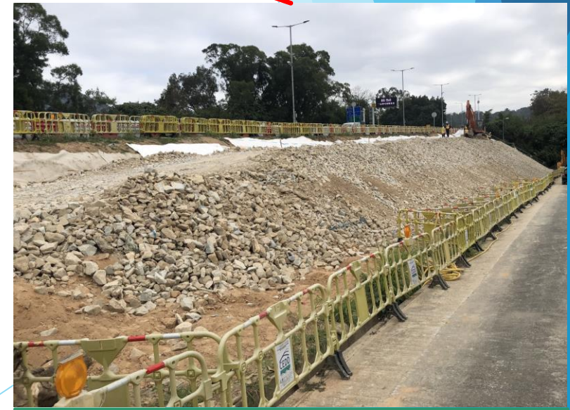
Rockfill Slope at Ch. 0 - 110 in progress
