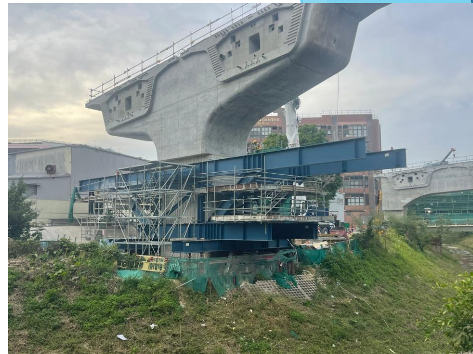
C4-02 Dismantling of temporary falsework in progress
