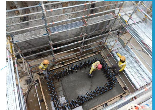
C1-02a pier kicker completed on 03/01/23
