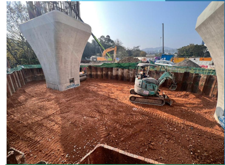
C1-03 Backfilling and sheet pile extraction in progress.
