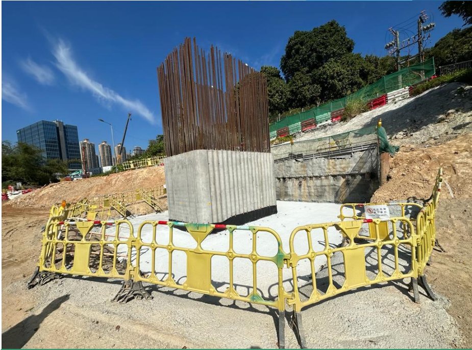
C3-02 cross head construction in progress
