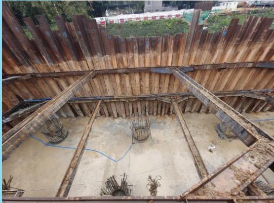
B1-01M Blinding Layer Casted
