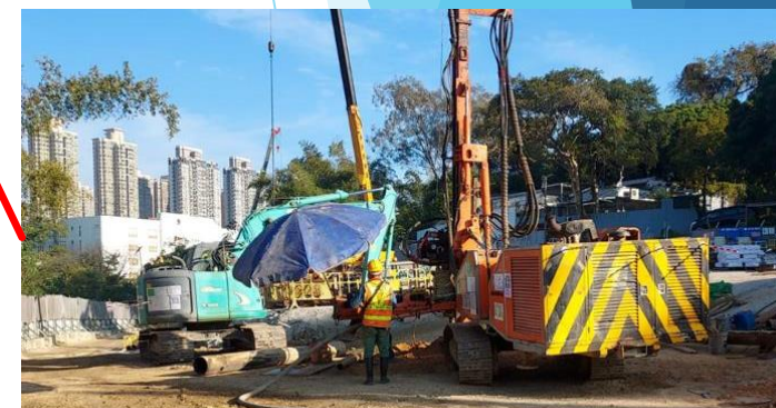
C3-01b pipe piling commenced on 05/01/23
