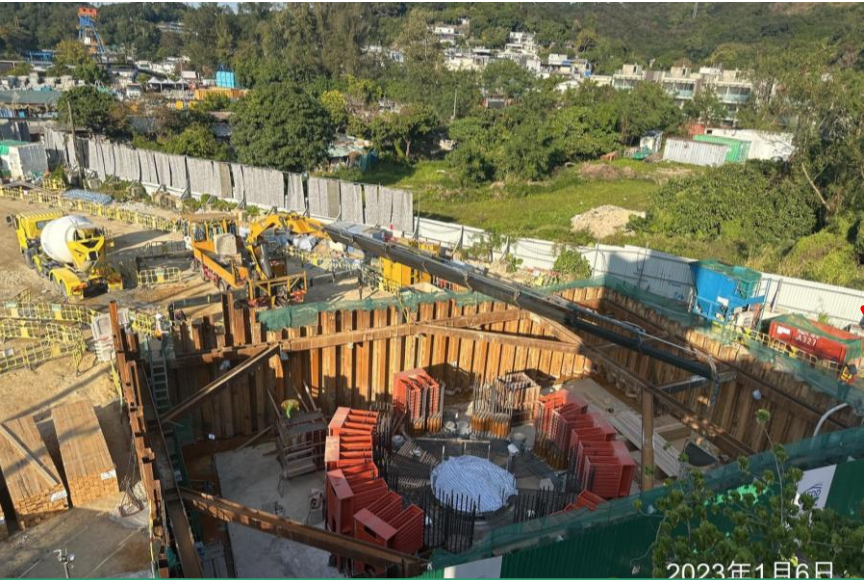
E2-01 primary reaction blocks completed concreting on 06/01/23.
