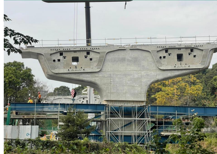
C4-02 Dismantling of temporary falsework in progress
