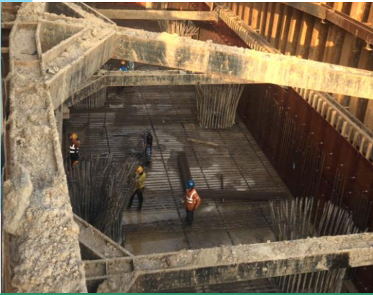
B1-01M Rebar Fixing in progress
