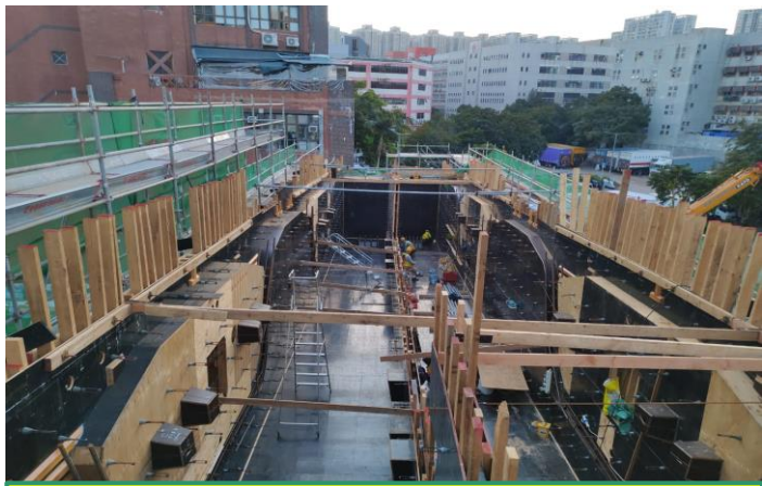
C3-04 portal beam side formwork completed on 22/11/22
