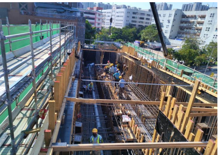
C3-04 MJ Portal Beam rebar fixing in progress
