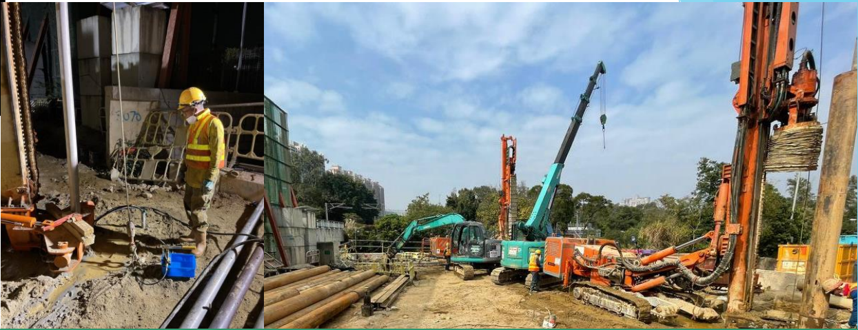
D2-01 pre-grouting works (within MTRC 6m Zone) in progress. Pipe piling (outside MTRC 6m Zone) in progress.
