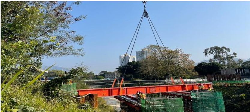
B1-02 portal beam construction in progress
