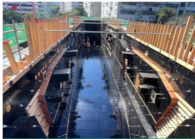
C3-03 portal beam side formwork completed on 06/1/23
