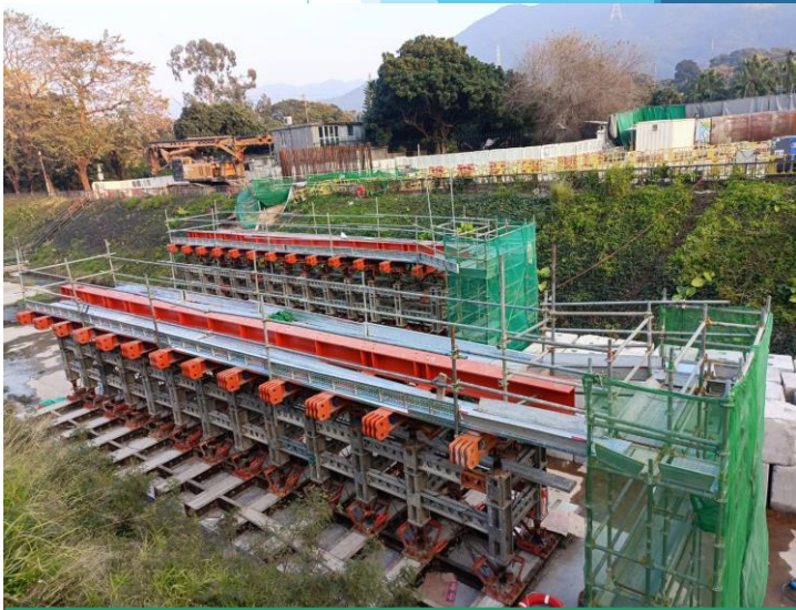
B1-02 Mega-shor tower for portal beam construction completed on 29/12/22
