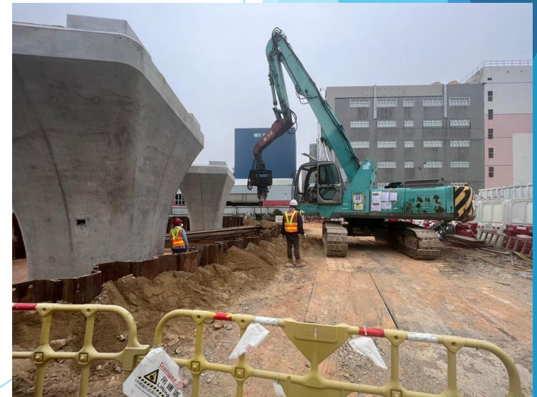
C1-04 Backfilling and sheet pile extraction in progress.
