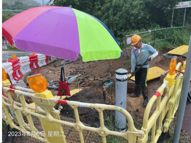
Cable duct laying & draw pit for traffic light , detection loop & street light
