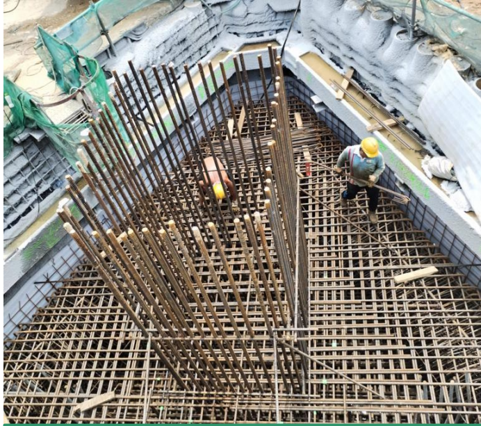
C2-04b pile cap rebar fixing completed on 03/06/23
