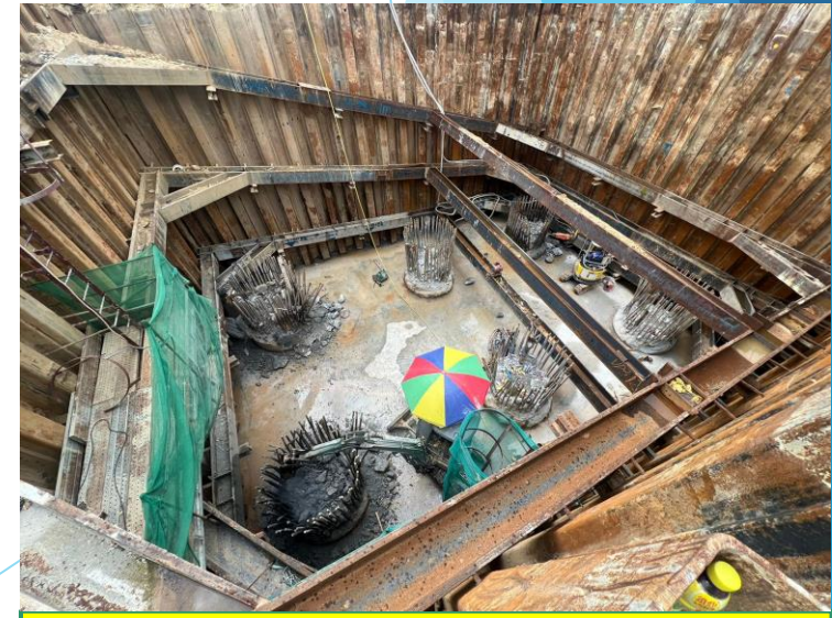
B2-03 Blinding Layer Cast, Bored Piles Head Breaking in Progress
