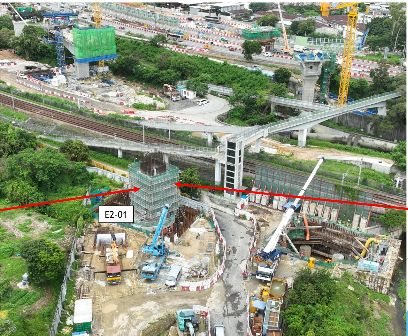
Dismantling of E2-01 steel mould at pier head (2 nd pour) completed on 07/06/23
