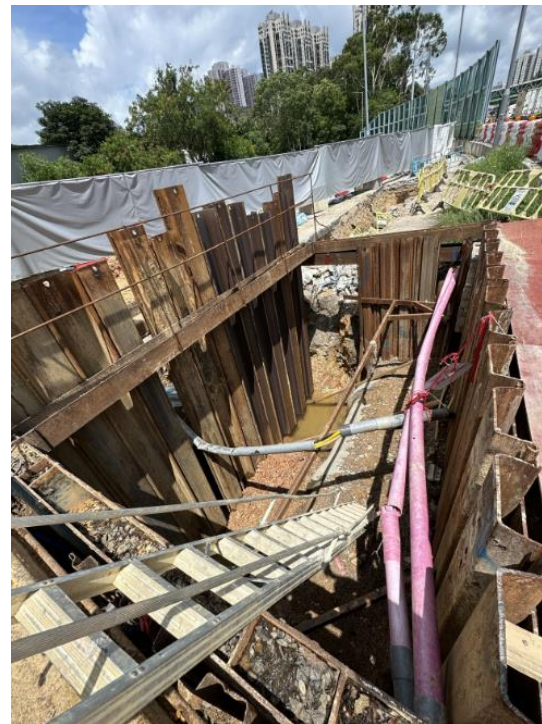
Construction work(ELS) of drainage manhole (FL9110)
