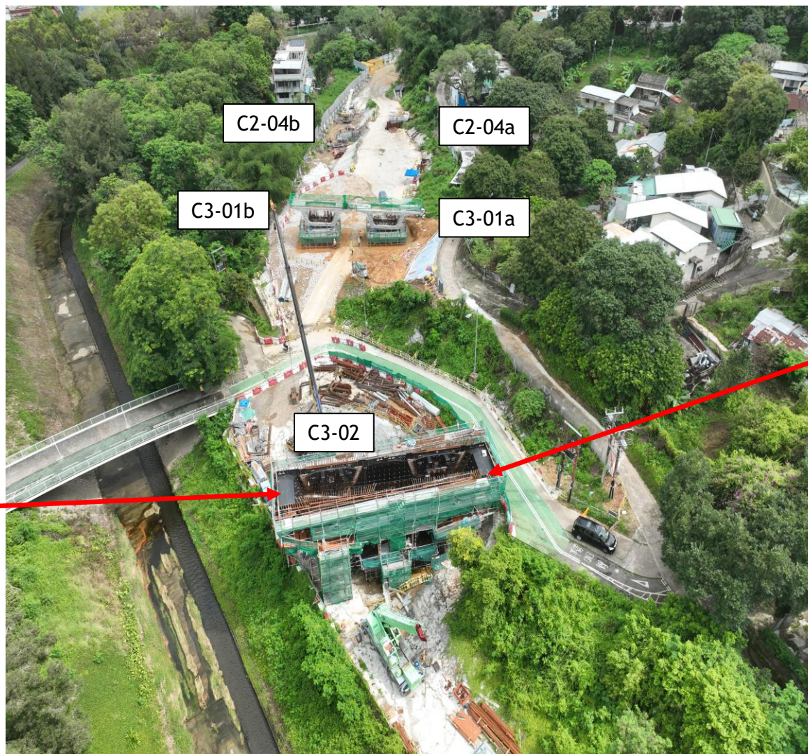
Rebar Fixing at C3-02 cross head construction in progress
