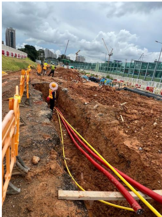
CLP 11kv cable laying (Between K.Kee Factory and Entrance of HKY)
