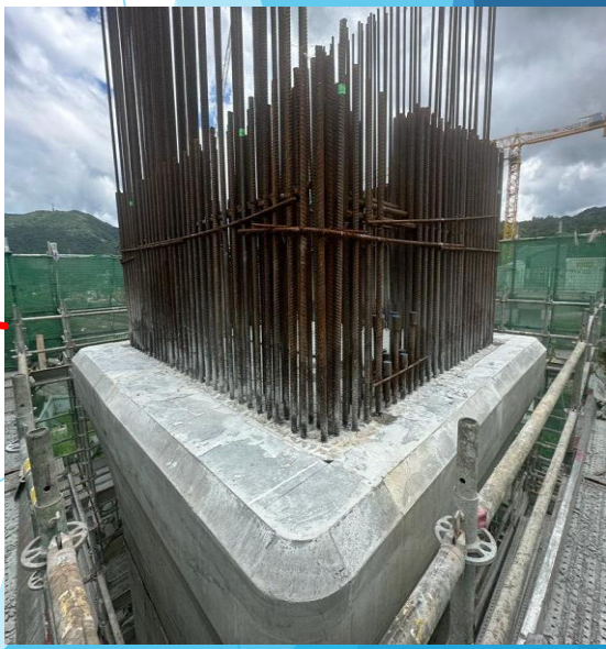
Dismantling of E2-01 steel mould at pier head (2 nd pour) completed on 07/06/23
