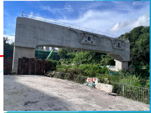
C3-03 Portal Beam completed hand over to bridge team on 07/06/23
