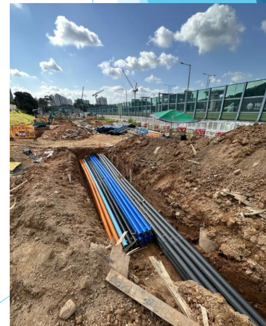
Ducts laying(Telecoms) (Near FS21)
