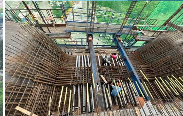
Rebar fixing at S07 segment (Lower Chainage) in progress
