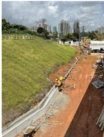
Construction work of U-channel at FS06
