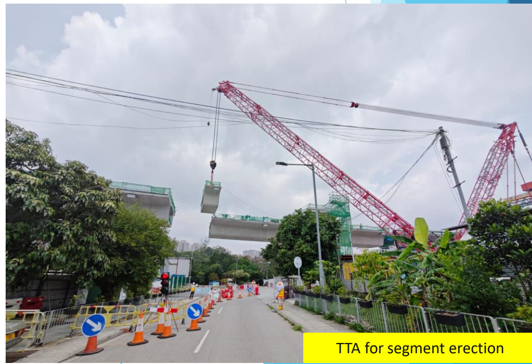
Lifting segment by crane
