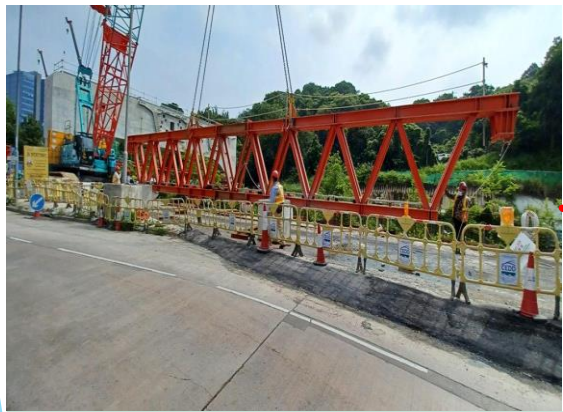
Dismantling of truss at C3-03 Portal Beam completed on 19/05/23
