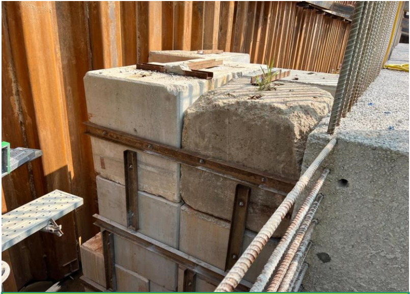
Concrete Block Retaining Wall Installation Completed
