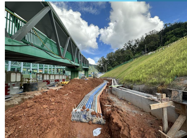
Ducts laying(Telecoms) (Near FS06)
