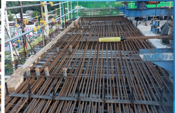
Rebar fixing at S05 segment (Up Chainage) in progress
