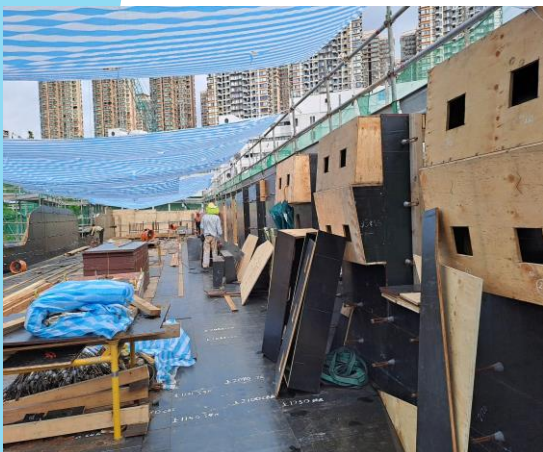
Side formwork at B1-02a portal beam in progress
