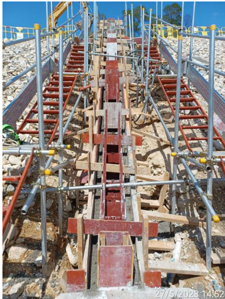
Construction of stepped channel at CH30
