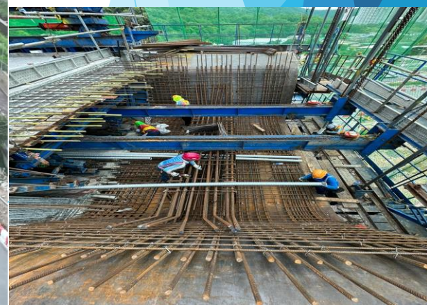
Rebar fixing at S07 segment (up Chainage) in progress
