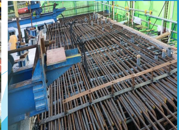
Rebar fixing at S05 segment (Down Chainage) in progress
