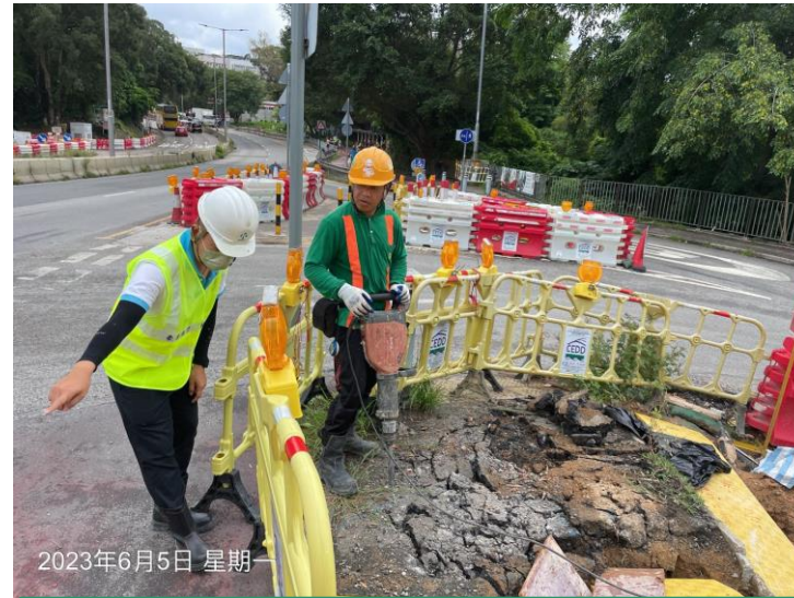
Breaking of existing footpath for cable duct laying for traffic light
