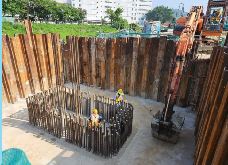
B2-02 Cap Concreted, 1 st & 2 nd layer of strut removed
