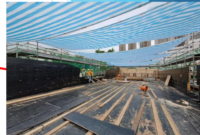
Soffit formwork at B1-02 portal beam completed on 01/06/23
