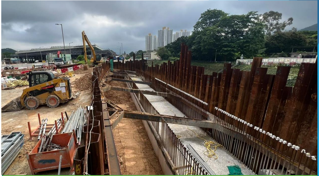
Backfilling in Progress
