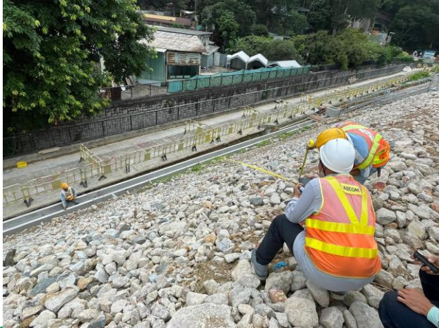
Rockfill slope works completed
