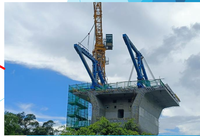
Main frame erection completed on 10/06/23
