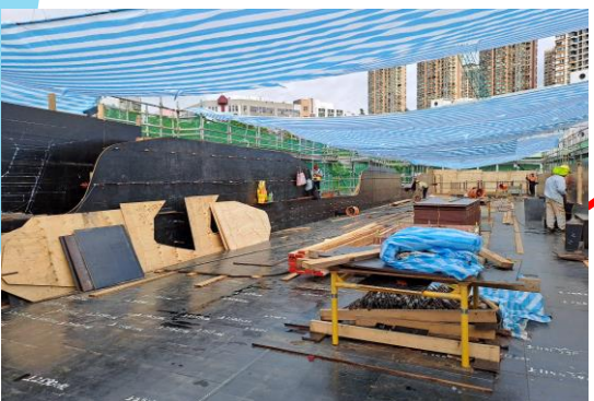
Segment kicker formwork at B1-02 portal beam in progress
