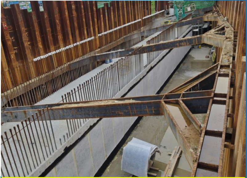
Bitumen Painting & geotextile installation completed
