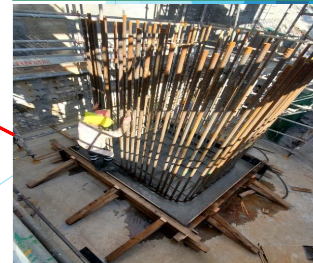
C2-04b pier kicker completed on 09/06/23
