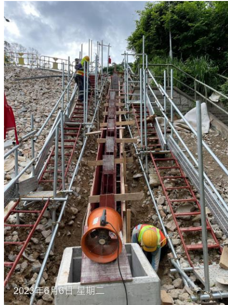
Construction of stepped channel at CH0
