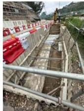
1" and 2" circuit completed. Backfilling work of joint bays are in progress.
