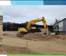
Laying sub-base layer (CH235 - CH290)
