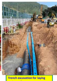
Trench excavation for laying water main
