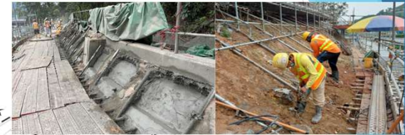
1. FS 04 - Soil Nail TSW 1138 (R15) ES: 01/11/22 EF: 04/05/23 LS: 19/05/23 LF: 16/06/23 • Digging work of soil nail head in progress • Concreting of soil nail head in progress
