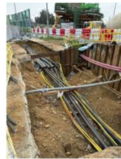
Removal work of existing CLP132Hv cable for gas connection work and construction work of drainage manhole (FL9110)
