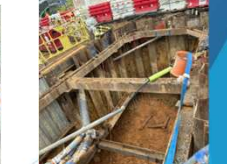
Trench excavation for laying DN1200 (drainage) • (Between FL9104A and FL9104B)
