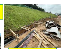
Construction work of U-channel at FS06
