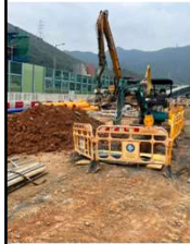
Excavation work of CLP 11kV joint bay for cable laying
