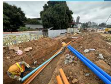
Ducts laying (Telecoms) (Between FS20 and FS20A)
