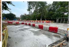
Concrete paving of new Wo Hop Shek Village entrance (Run-in)
