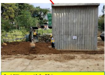
Backfilling to +10.3mPD in progress.
