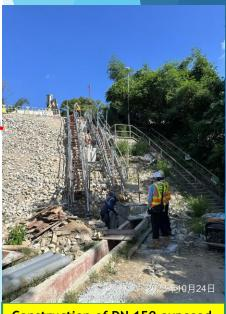
Construction of DN 150 exposed pipe concrete footing in progress.
