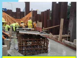
Abutment wall (2nd pour, part 2) concreted on 21/10/23, bearing plinth cast on 30/10/23
