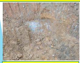
Inspection pit was carried out to verify the depth of WSD sleeve pipe
