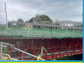
Temporary falsework support at C1-02a in progress
