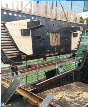
Side formwork for C2-01 cross head completed on 10/11/23
