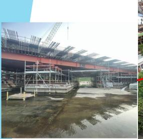
Dismantling of steel beam at B1-02 portal in progress
