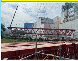
Truss assembly for C1-02 portal beam construction completed 26/10/23
