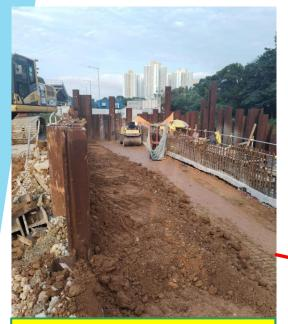
Backfilling to +10.8mPD (road side) completed on 27/10/23
