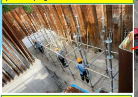
Falsework erection for B2-02 cross head construction in progress
