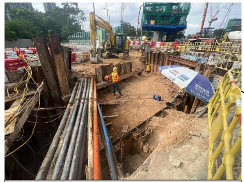
Excavation for 2xD1200 Stormwater Pipe in Progress. Target 30/11 reach Formation.
