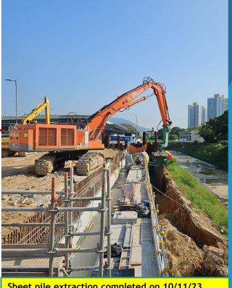
Sheet pile extraction completed on 10/11/23
