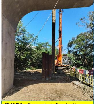
C2-02 ELS cofferdam sheet pile extraction completed on 24/10/23
