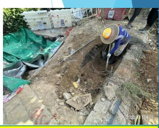
Trial pit for 900mm dia. drain pipe and manhole SMH\_FL8701 in progress.
